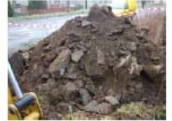
TP4 quarried stone dump from fill of trial pit
