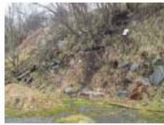
Area of TP4 stone dump (2)
