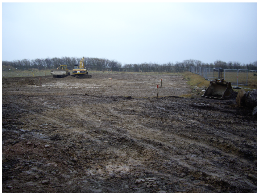
Plate 1: Initial Soil Scrape, facing east
