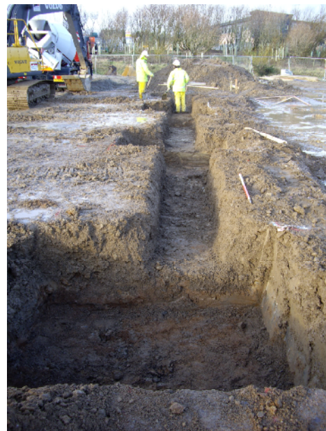
Plate 3: Pits 22, 21 and 20 with adjoining strips, facing west
