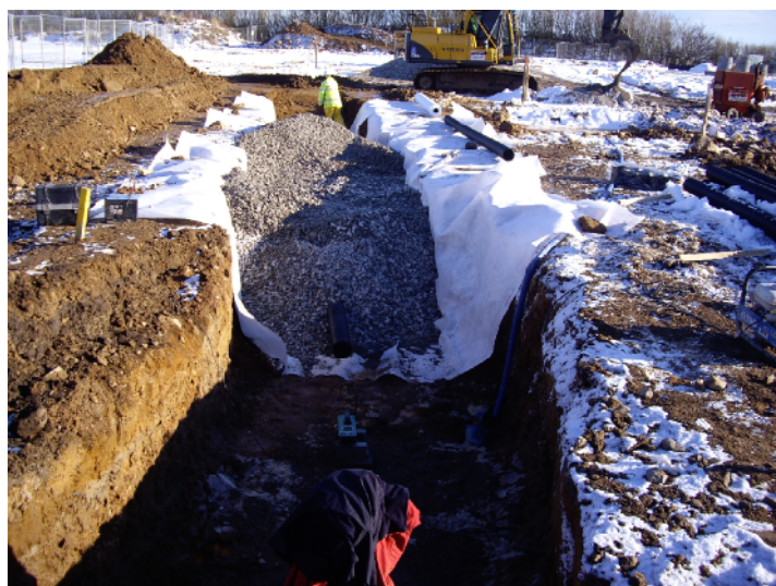
Plate 5: Foul Drain Channel, facing east
