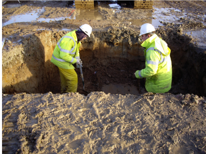
Plate 4: Lift Shaft Pit, facing east
