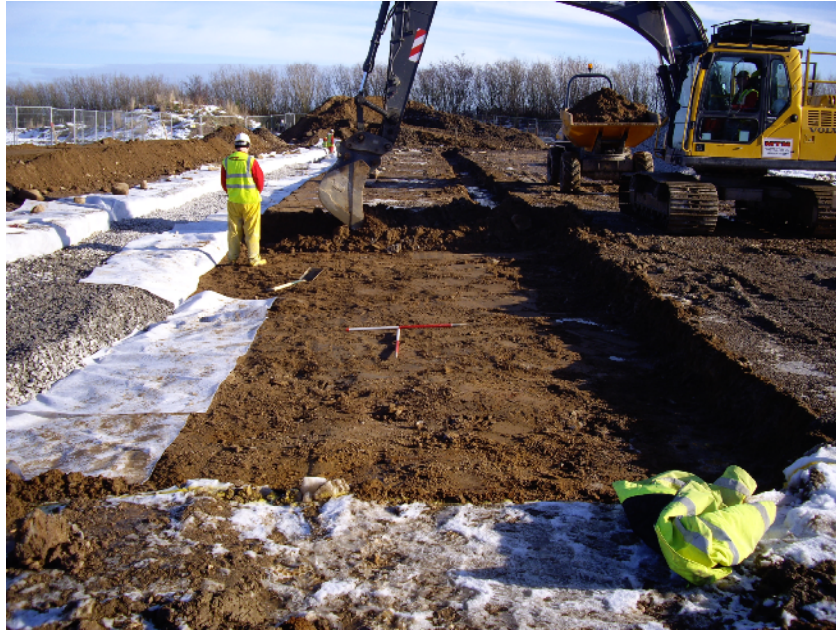
Plate 7: Car Parking Area under excavation, facing east
