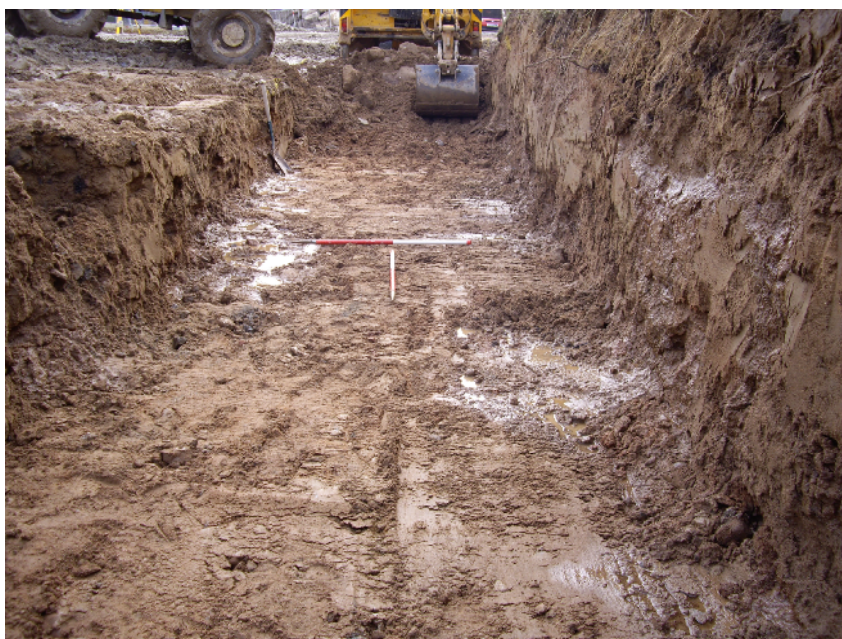
Plate 6: Filter Drain Channel, facing south
