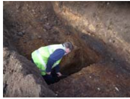
Tr 2 AH excavated (5)
