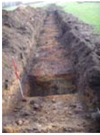
Tr 2 AH excavated (4)
