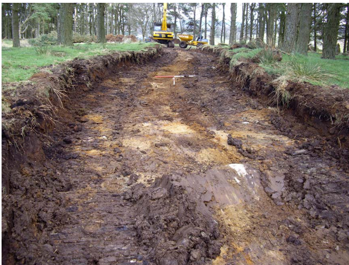
Plate 1: View of easternmost part of excavation facing west
