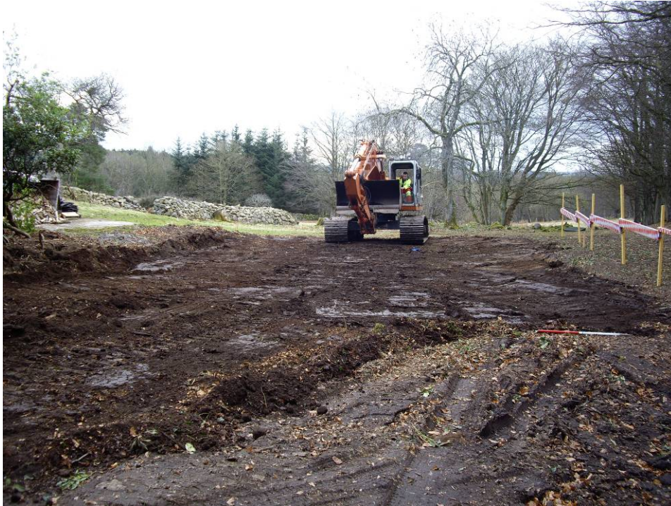
Plate 2: Soil Scrape of workshop footprint area, facing east
