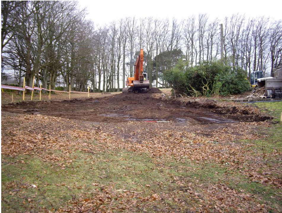
Plate 1: Soil Scrape of workshop footprint area, facing west
