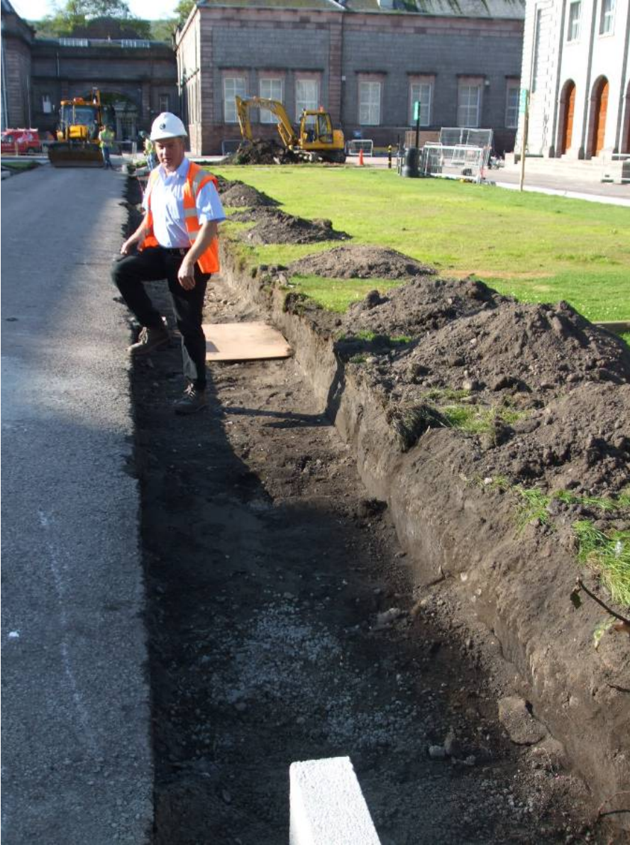
Trench along the edge of the grass for fencing
