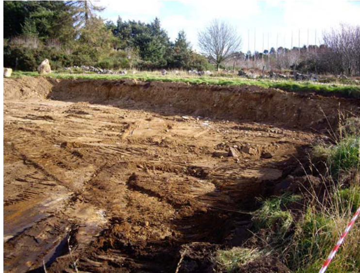
Plate 2: Levelling of storage buildings area, facing south
