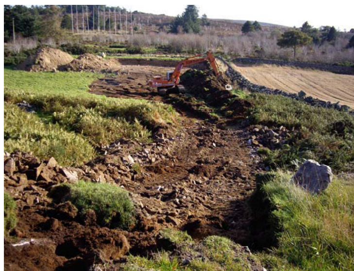
Plate 4: Preparation of access track, facing south
