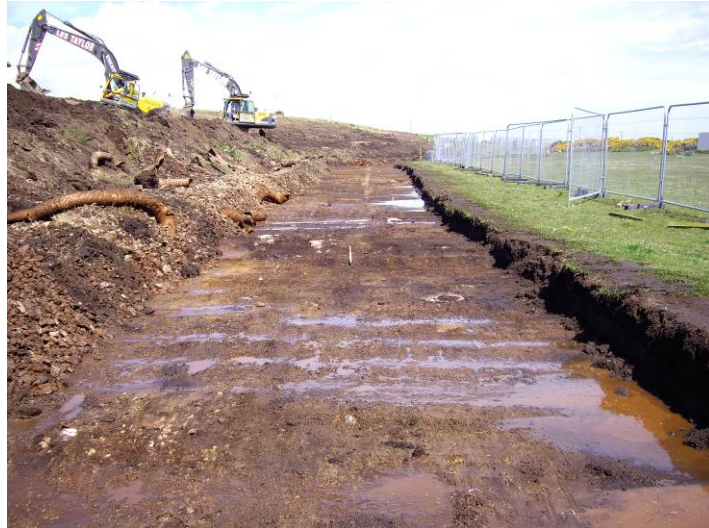
Plate 1: General view of topsoil strip, south-eastern area, facing north-east
