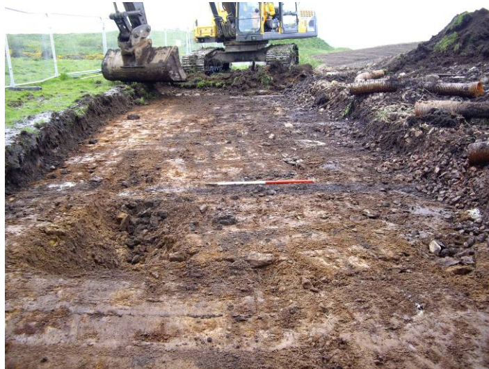
Plate 4: Feature 3 facing north-west
