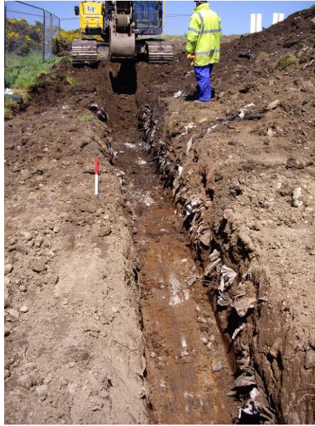
Plate 6: General view of topsoil strip extension, facing north
