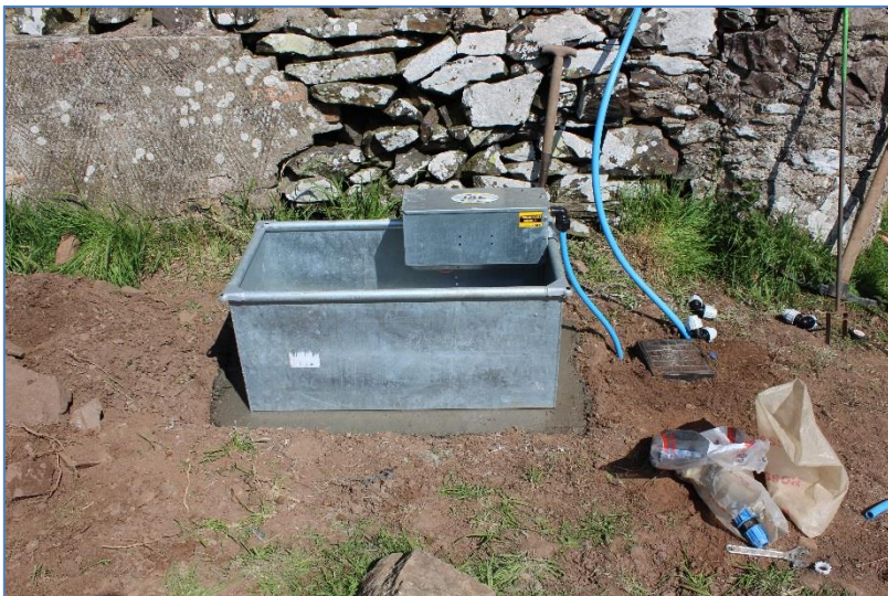
Figure 5: After water trough base and new toby installation
