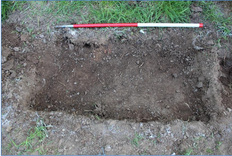
Figure 3: Post-excitation of trench for trough base
