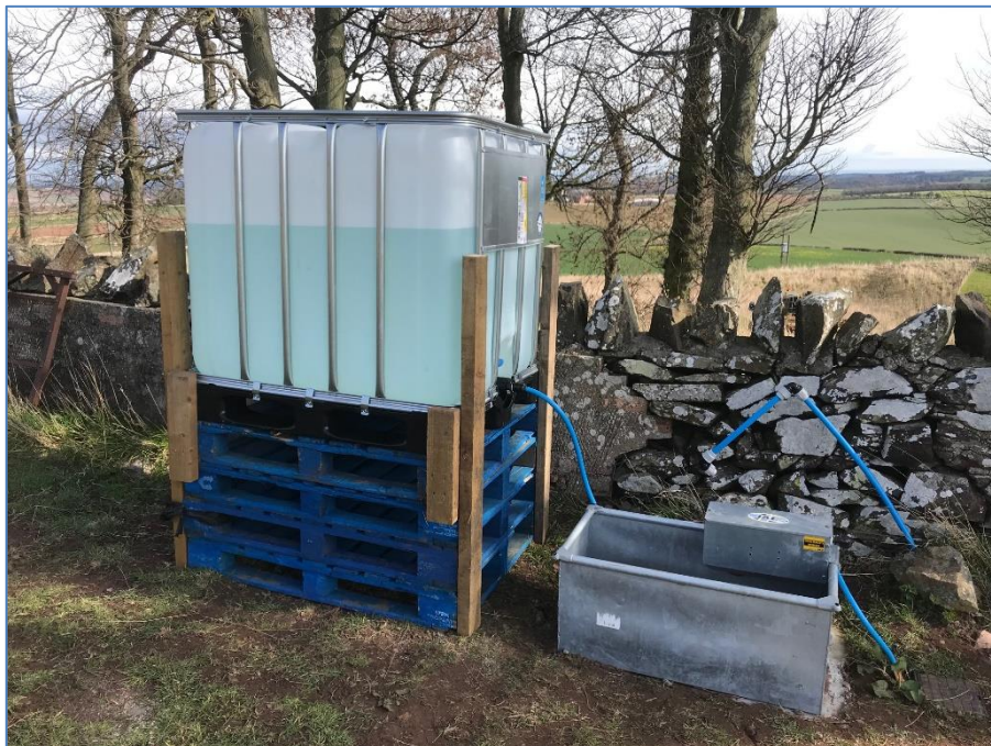
Figure 6: Water tank and trough following installation
