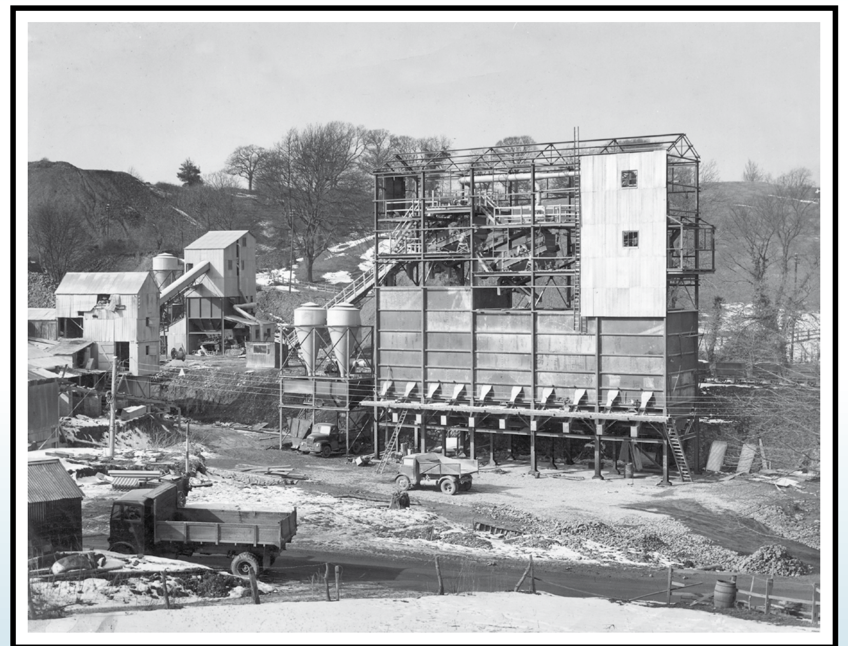
▲ This building is where quarried material is processed into forms suitable for road building and construction. It was built some time between the 2nd World War and 1965. The products from this process would be funnelled into the back of road lorries as opposed to railway wagons in the past.
