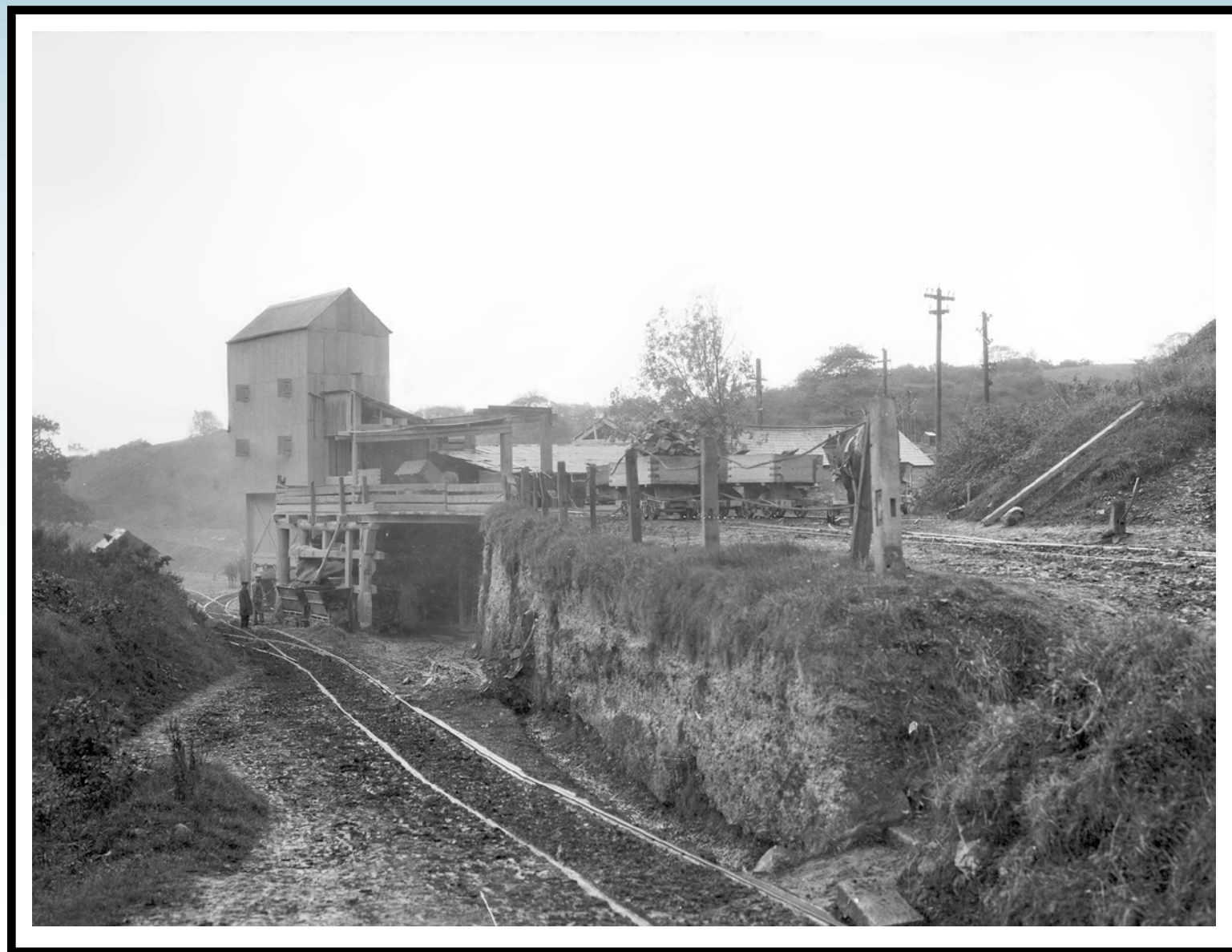
◀ This building contained machinery which sorted the quarried material into different grades or sizes.
