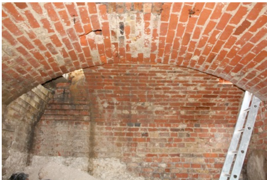
Figure 7: End wall of chalk lined structure facing south west
