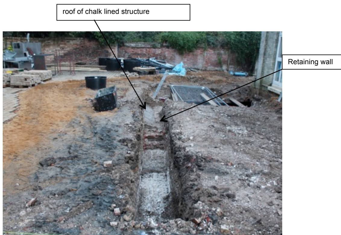
Figure 8: Trench showing chalk lined structure and retaining wall
