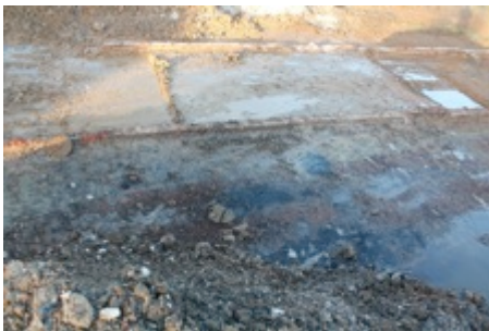
Figure 11: East facing view of brick foundations
