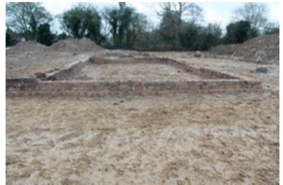
Figure 24 North facing view of Mill Corner
