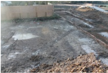
Figure 9: South East facing view of brick foundations and 1911 kiln location
