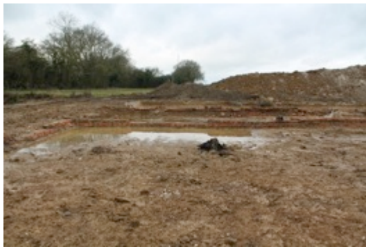
Figure 25: East facing view of Mill Corner Farm 1 of 4
