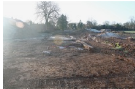
Figure 8: South facing view of brick foundations
