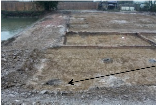
Figure 45: Posthole [35] location within Mill Corner Farm
