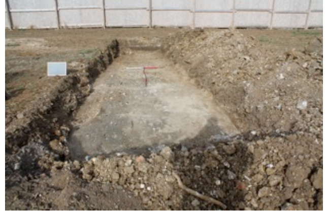
Figure 9 South facing view of Trench 2
