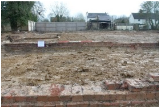
Figure 41: West facing section of internal wall F(68) internal wall F(56)
