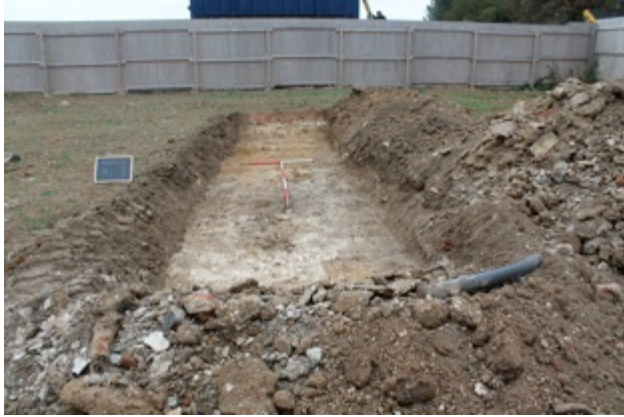
Figure 8 South facing view of Trench 1
