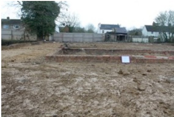
Figure 39: West facing section of external wall F(55) wall F(68)
