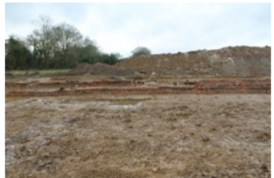
Figure 26: East facing view of Mill Corner Farm 2 of 4
