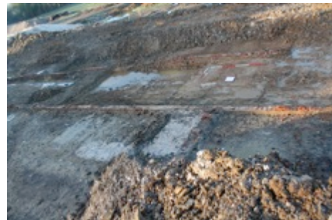
Figure 10: East facing view of brick foundations
