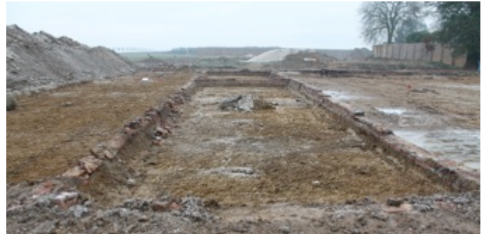
Figure 17: South facing view of Mill Corner Farm 2 of 4
