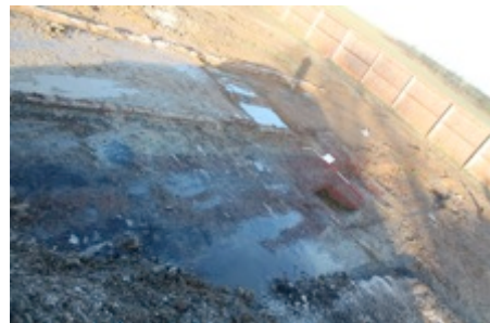
Figure 12: North East facing view of brick foundations
