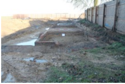
Figure 7: North facing view of brick foundations
