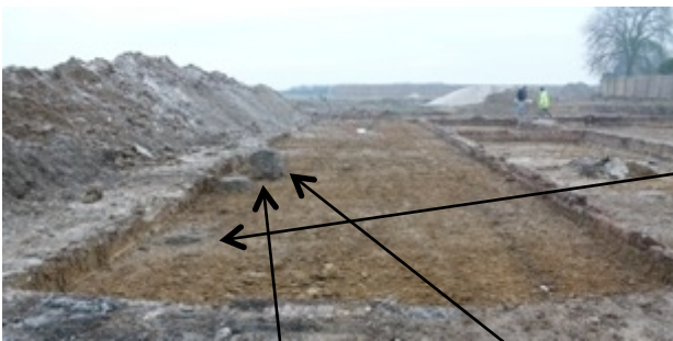
Figure 47: Posthole/pit [47] location within Mill Corner Farm
