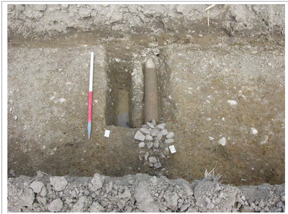
Plate 2: View of excavated land drains within Trench 1, Scale 1x1m
