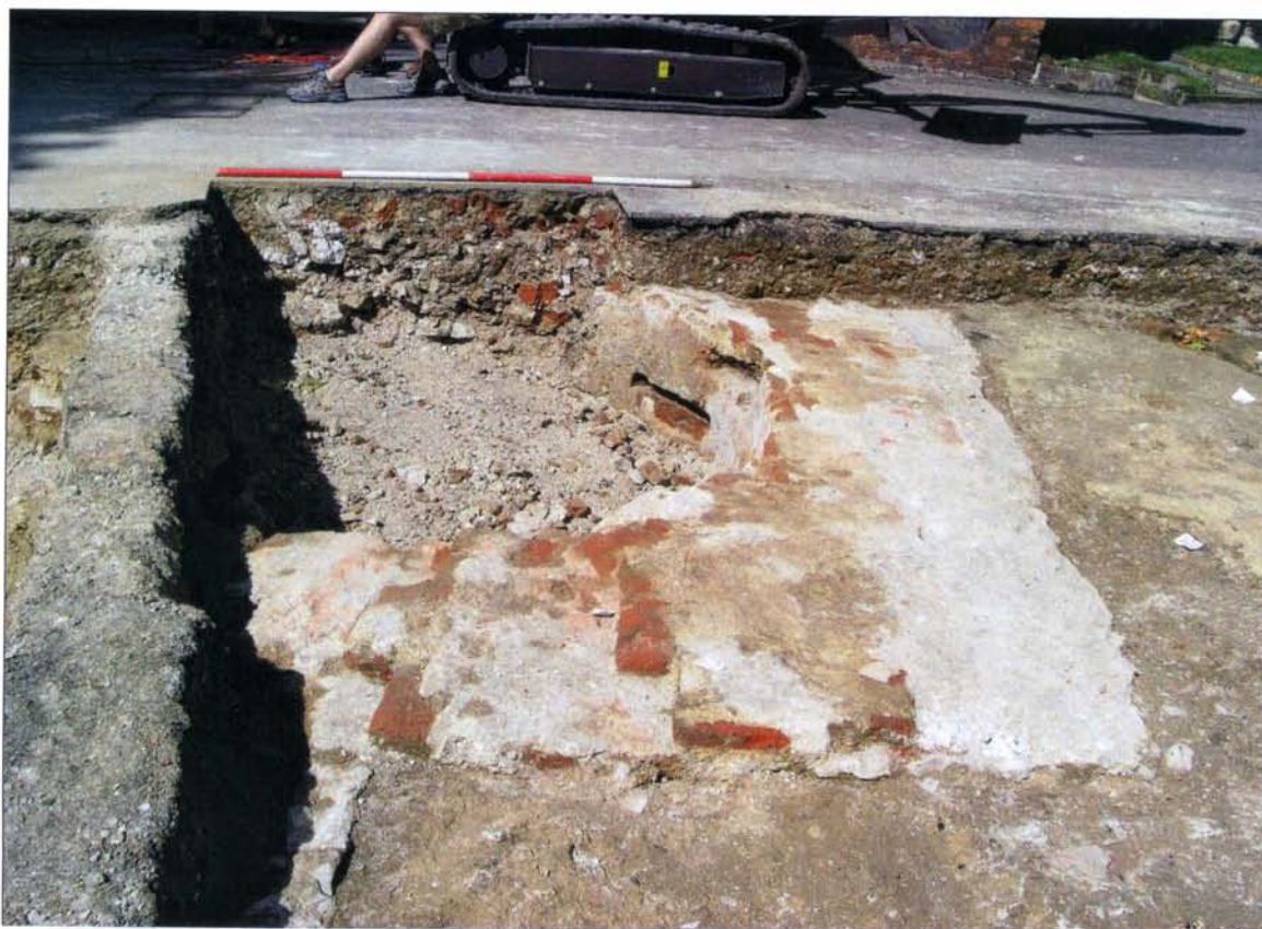
Plate 14. Trench 1. Context no 104 - Dentons Commons spiral staircase. Looking northwards.
