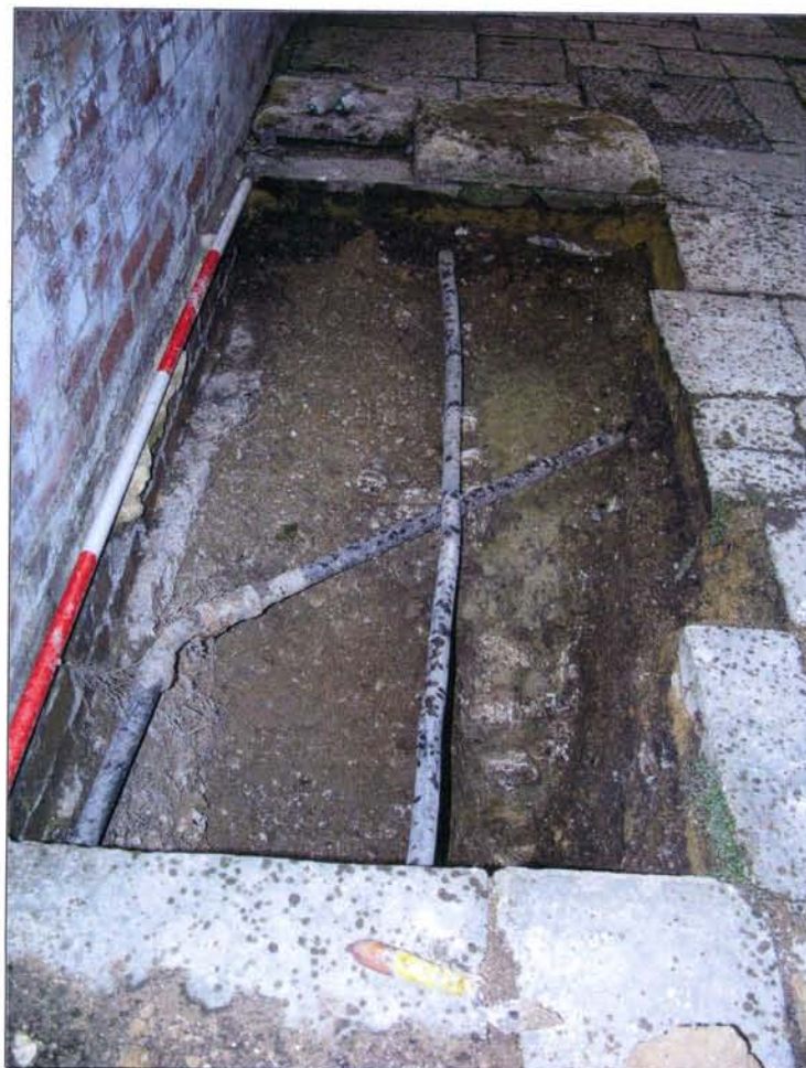
Plate 30. Trench 4. Stone slabs lifted and bedding removed.
