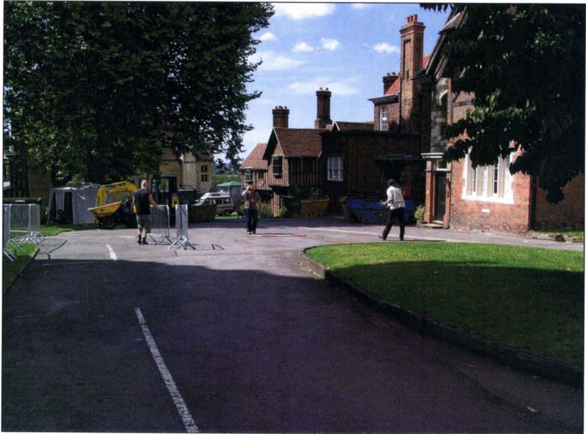
Plate 1. Area of excavation. Looking west.
