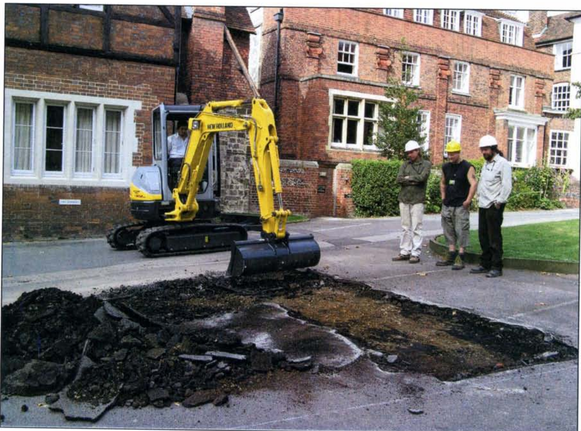
Plate 4. Initial removal of tarmac for insertion of Trench 1.
