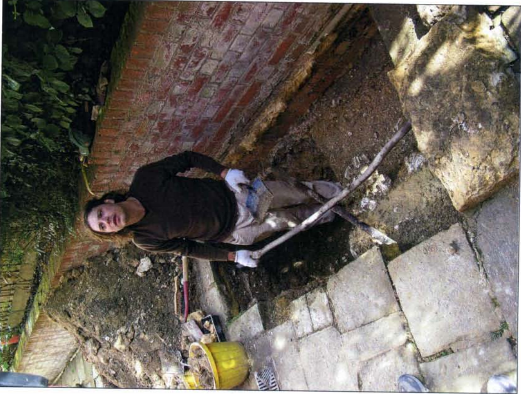
Plate 31. Trench 4. Slot put in trench to get profile through wall robber trench and chalk/clay surface.
