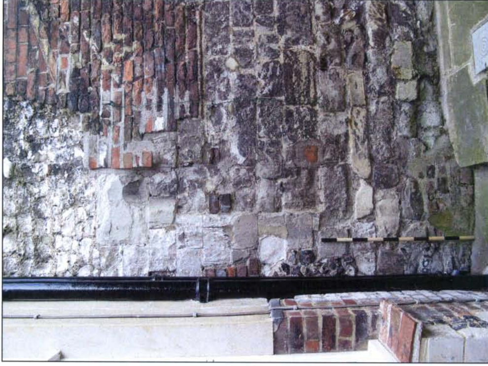
Plate 38. Evidence of possible former doorway and earlier wall at rear exterior of Chorister Lodgings No: 25. Alongside northern curtain wall.
