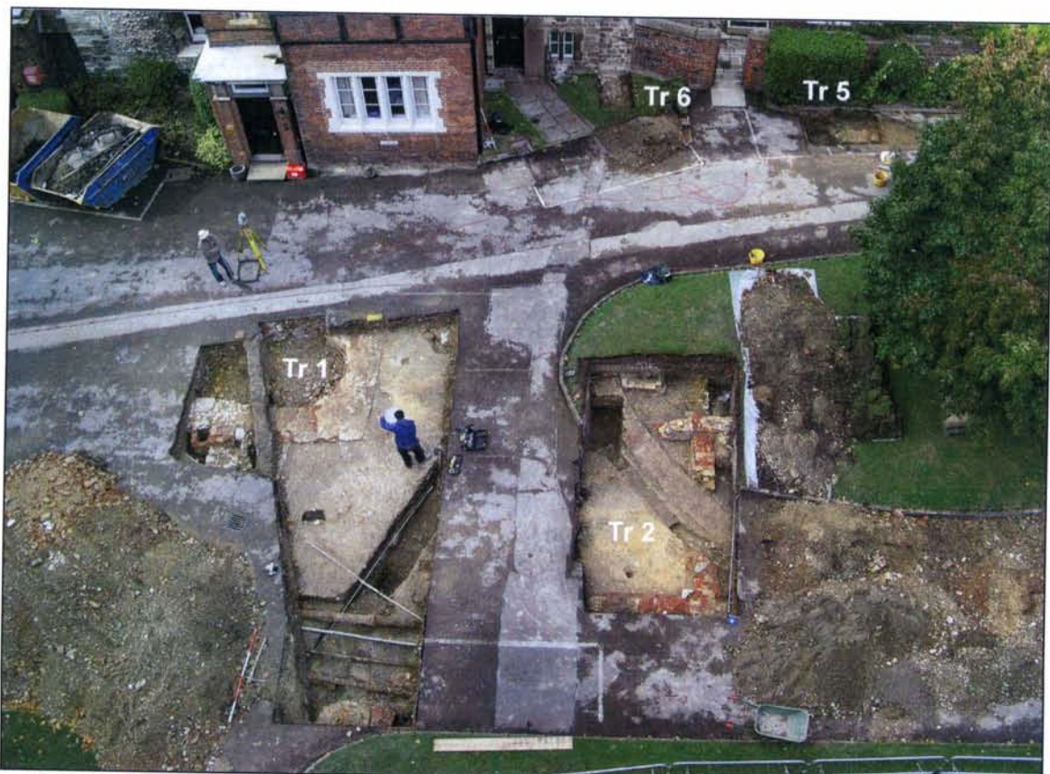
Plate 6. Aerial view of Trenches 1, 2, 5 and 6 following excavation. Taken from roof of St. Georges Chapel
