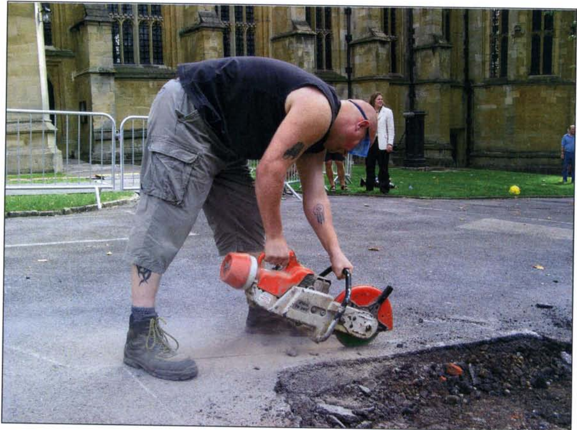
Plate 5. Cutting of tarmac for trench 1 Looking south..
