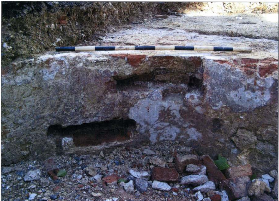
Plate 20. Trench 1. Detail shot showing slots for wooden stairs in Dentons Commons spiral staircase. Looking eastward.
