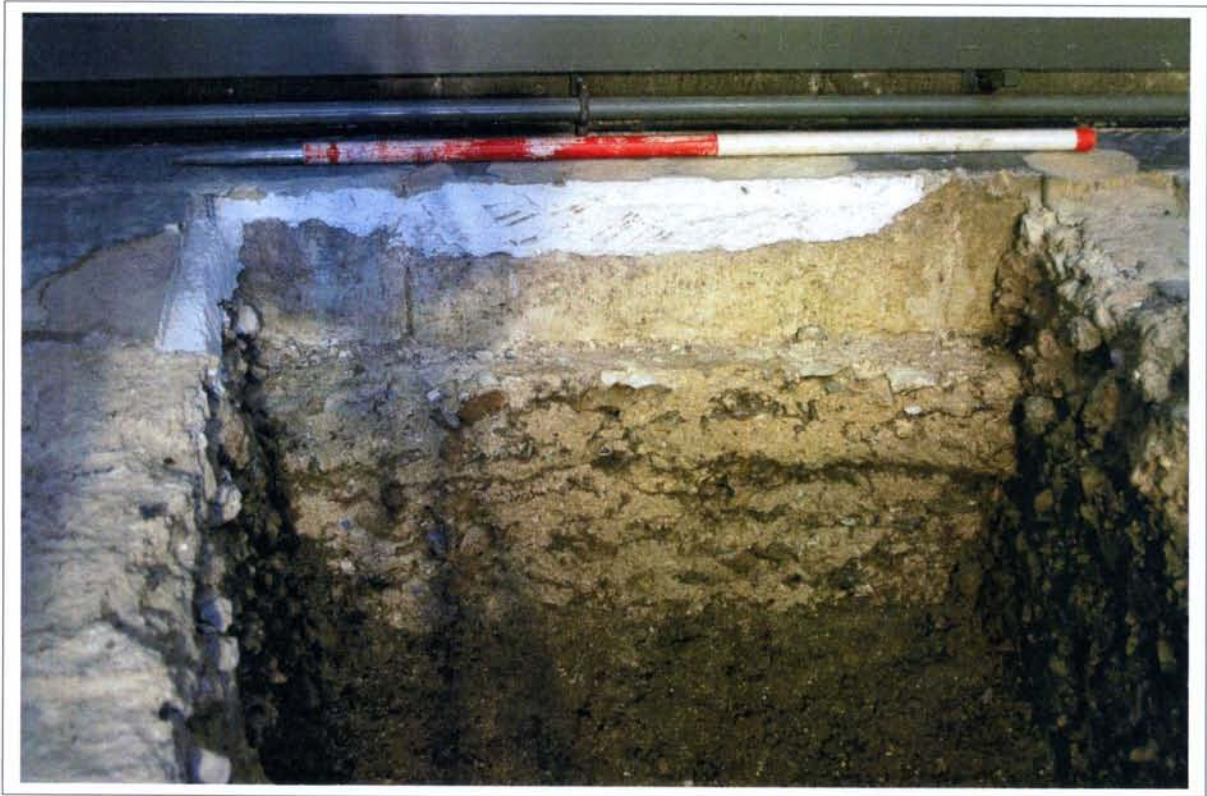
Plate 7: View of south wall and footing, Scale 1x1m
