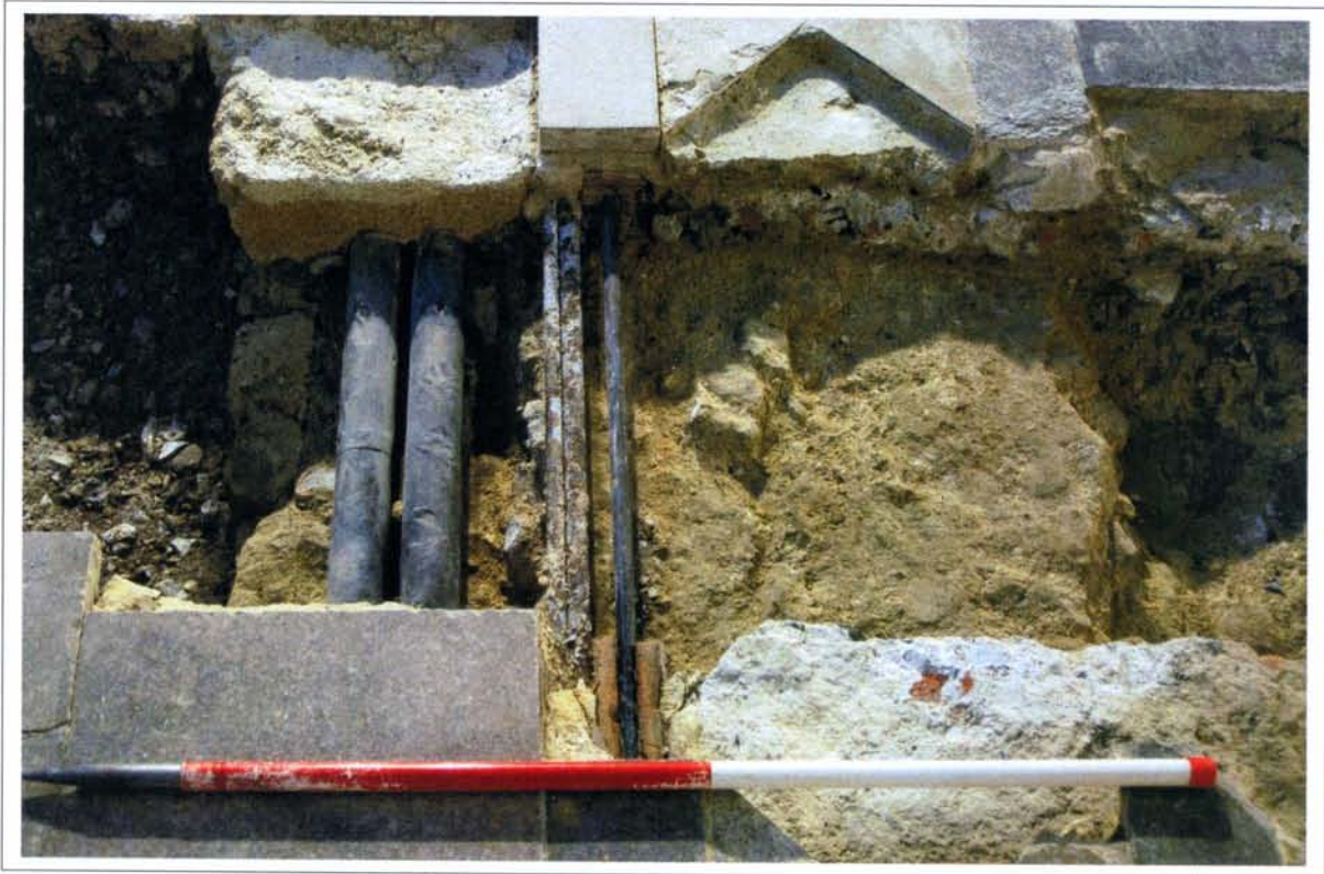
Plate 25: View of pipes on south side, Scale 1x1m
