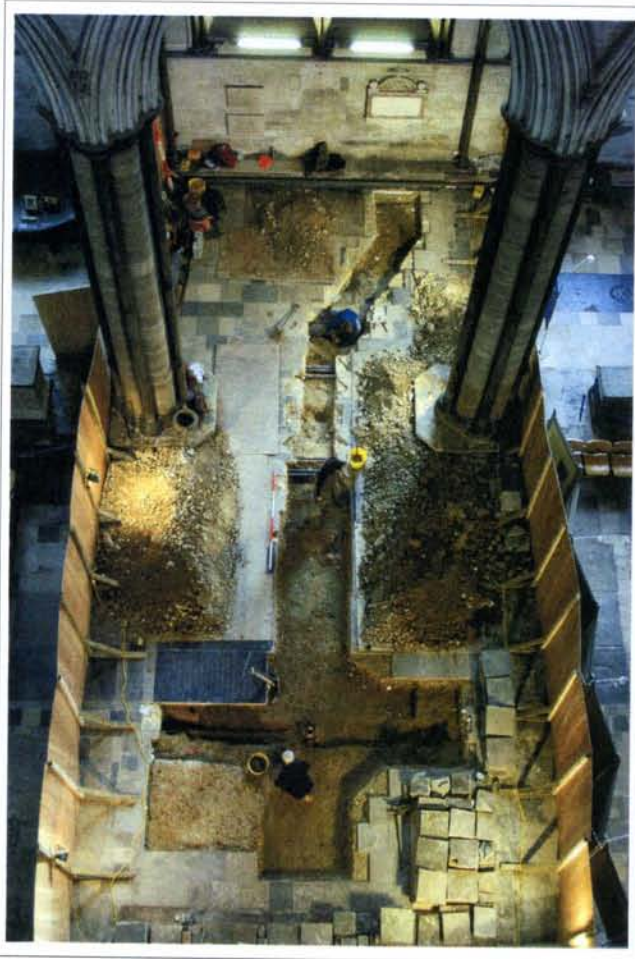
Plate 19: View of excavated 19th century levelling, Scale 1x2m
