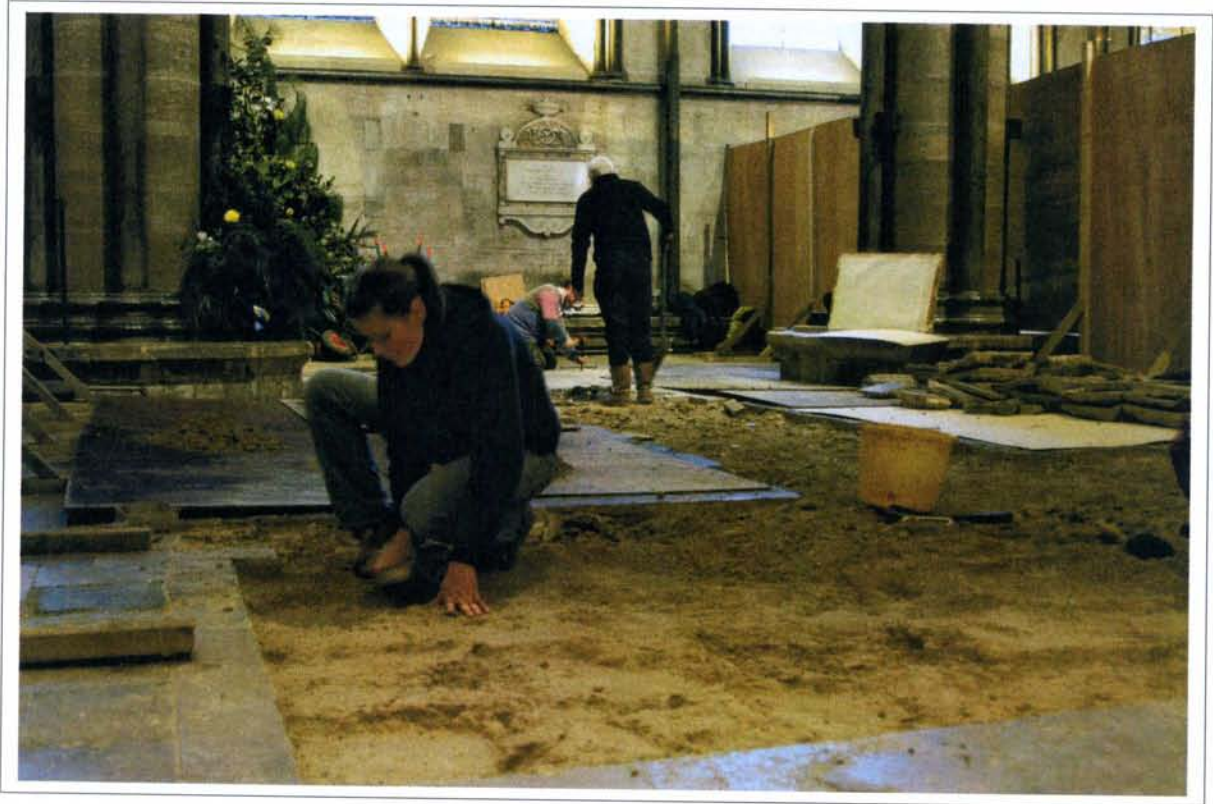
Plate 21: View of mortars being excavated
