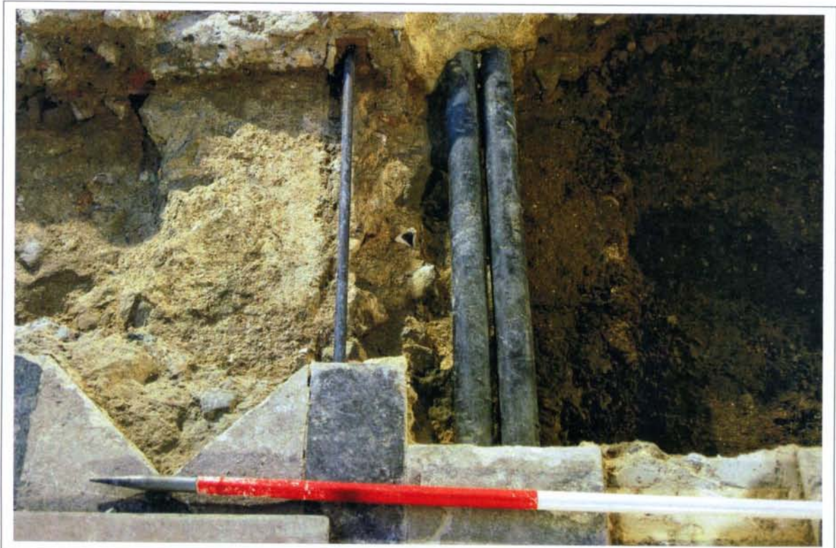
Plate 26: View of pipes on north side, Scale 1x2m
