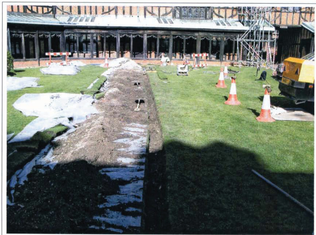
Plate 3: View of trench across Horseshoe Cloister lawn, Looking north
