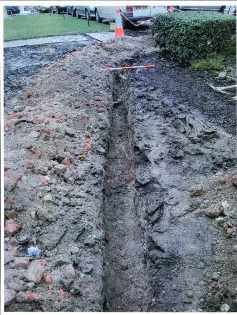
Plate 6: Example of rubble excavated on site of Dentons Commons building
