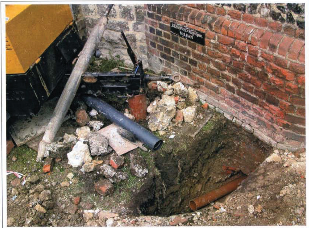
Plate 14: View of trench in area of Great Hall wall, Looking north
