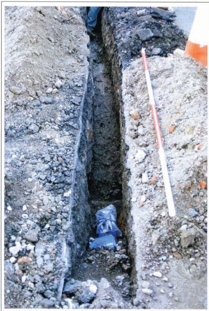
Plate 11: View along service trench Scale 1x2m, Looking west
