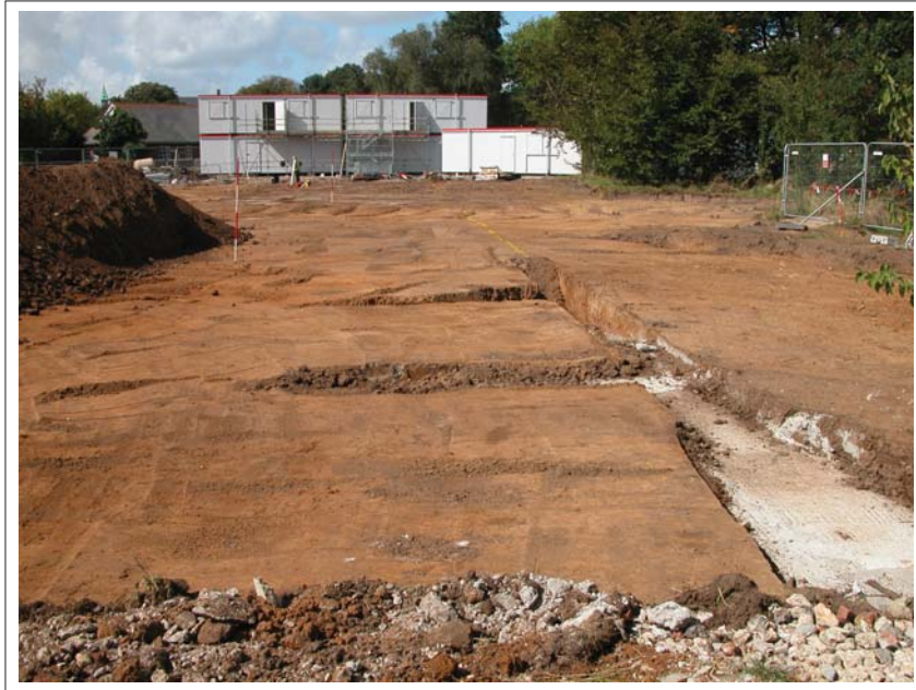
Plate 3 Northern Area after Foundation Trenching
