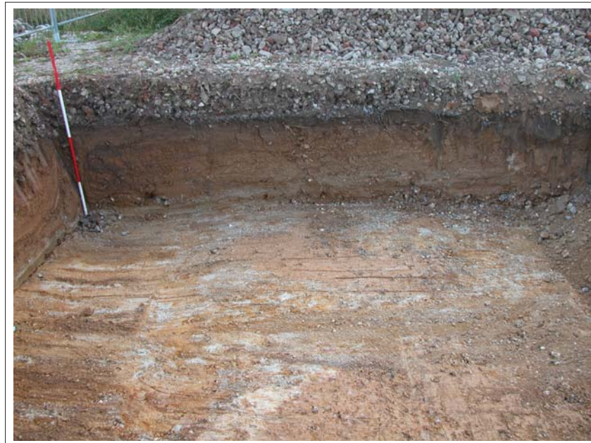
Plate 4 Soakaway at East of Site, Imported Hardcore
