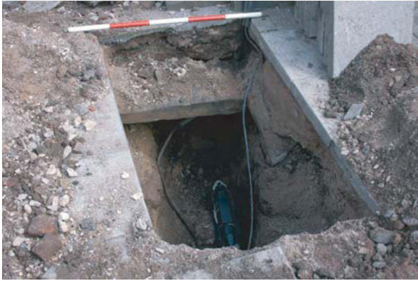
Trench 1, looking east, scale 1m
