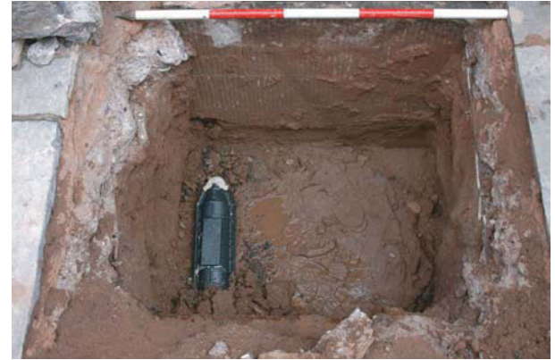
Trench 3, looking south, scale 1m
