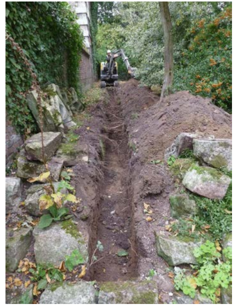
Plate 3 View of Intervention 8 looking north
