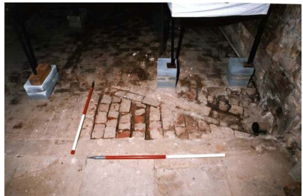
Plate 1 Location of undercroft sump pre-intervention
