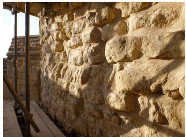
Plate 4 Herringbone masonry in the south curtain wall to the west of the Observatory Tower
