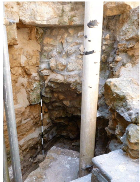
Plate 21 East Gate, blocked doorway in south bartizan turret
