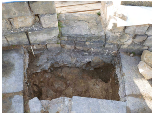
Plate 9 Test pit cut into the south curtain wall walk, east end
