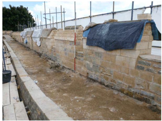
Plate 11 South curtain wall parapet wall-walk with modern surface removed
