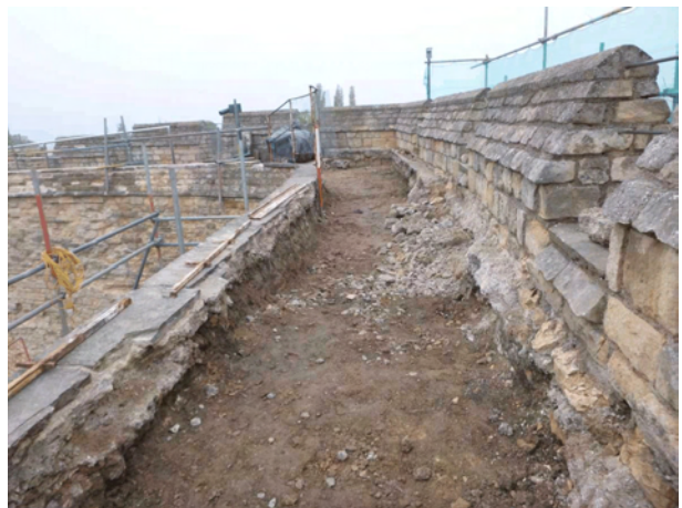
Plate 26 Medieval core-work exposed on north curtain wall
