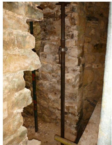
Plate 16 Unblocking of west chamber door opening
