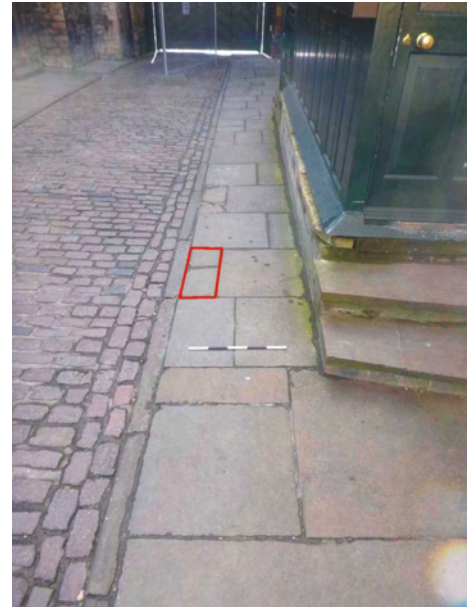
Plate 2 View of slab prior to replacement
