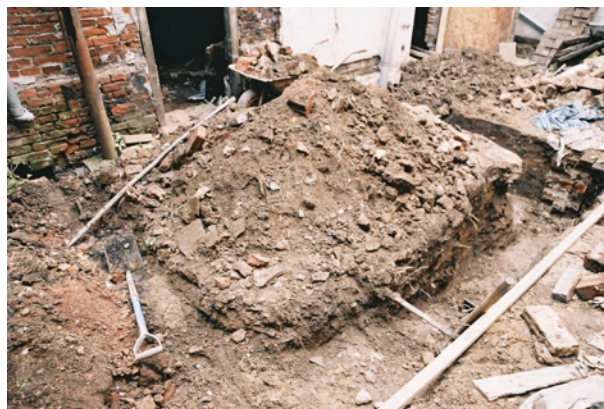
Plate 3 Excavated foundation trench to the rear of 2-4 Millgate
