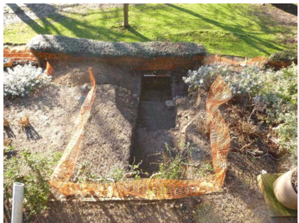
Plate 6 Intervention 25 looking south (scale 1.0m)
