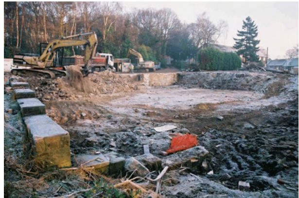
Plate 4 Basement foundation removal, looking northeast
