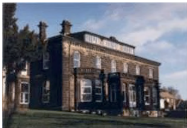
Plate 1 Iveson House, main facade
