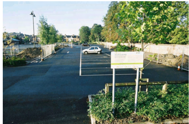
Plate 1 Site of Intervention 1 to 4
