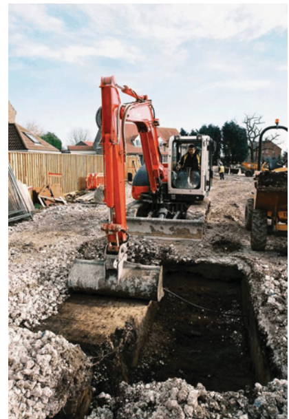
Plate 3 Manhole excavation
