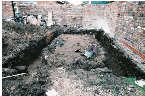
Plate 1 Foundation trench, looking west
