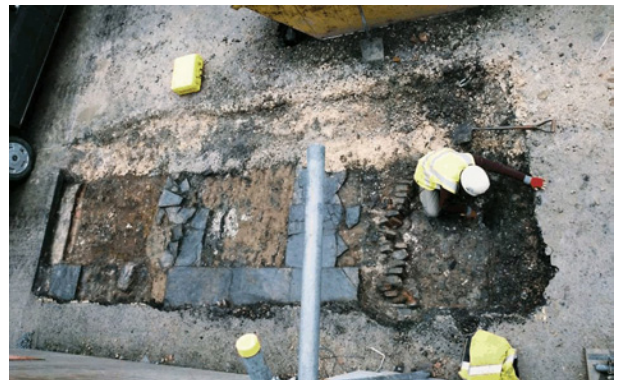
Plate 8 Structure 1 during excavation
