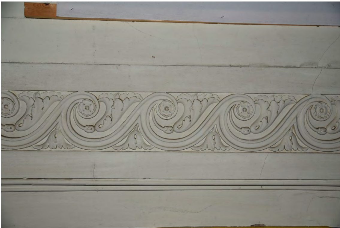
Plate E26 Detail of vestibule decorative plasterwork frieze, looking W (BRH204)
