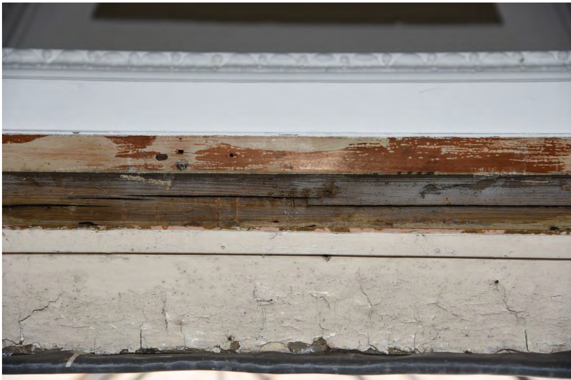
Plate E120 Lantern SW elevation – Carpenters' mark inside top of window frame = II (BRH066)
