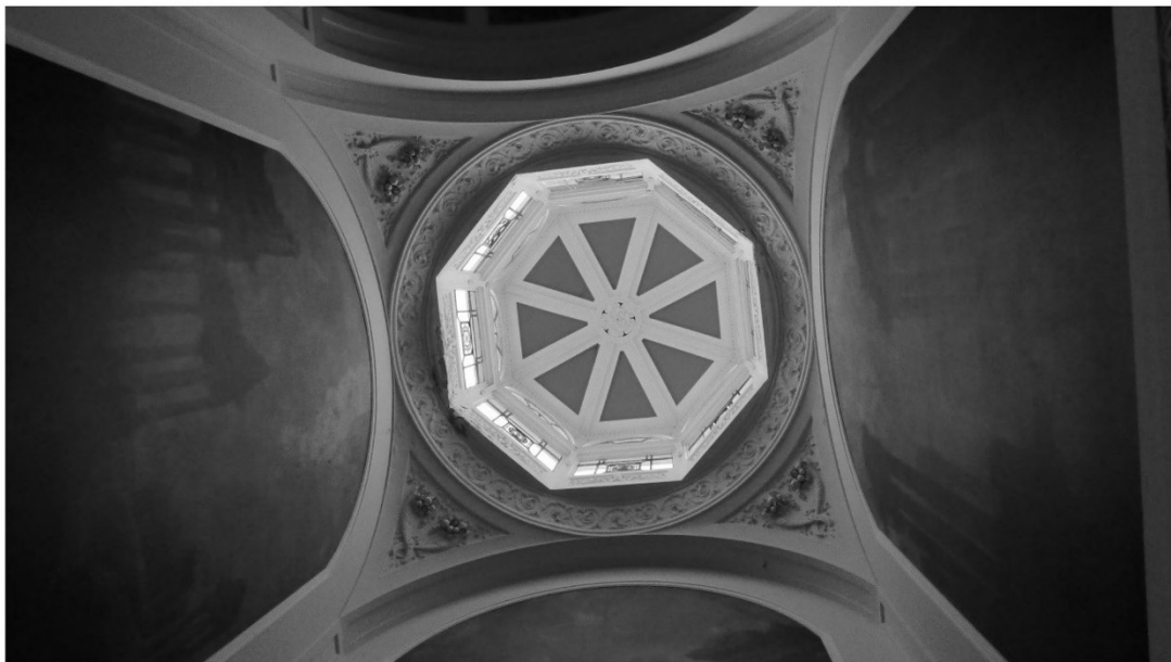
Figure 3 Internal view of the lantern © David Hunter /WYAAS
