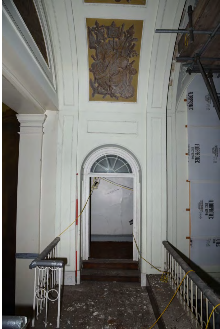
Plate E35 Vestibule passage from staircase, W elevation, looking W, scale 2.0m (BRH213)
