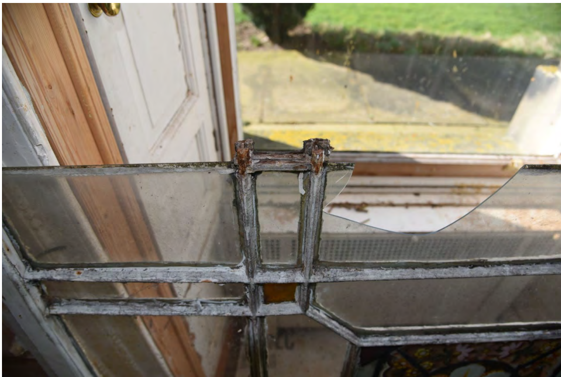
Plate E142 Detail of cast iron glazing bar (BRH180)
