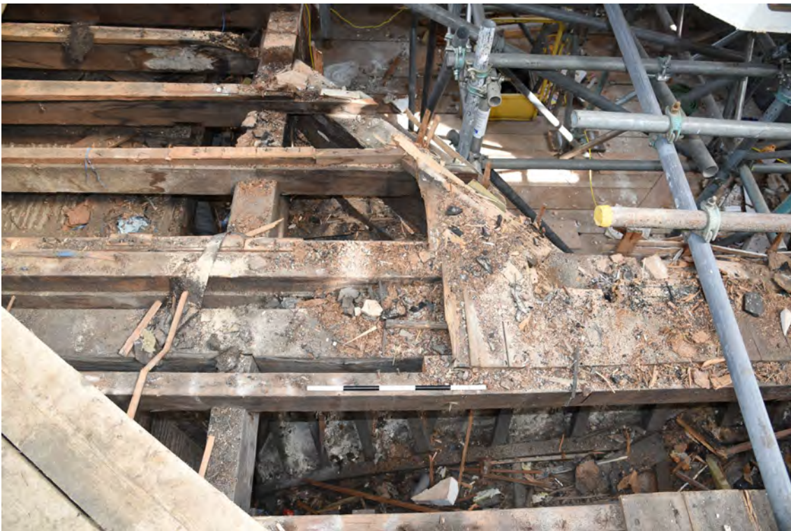
Plate E102 View showing roof construction SW pendentive, looking N (BRH139)
