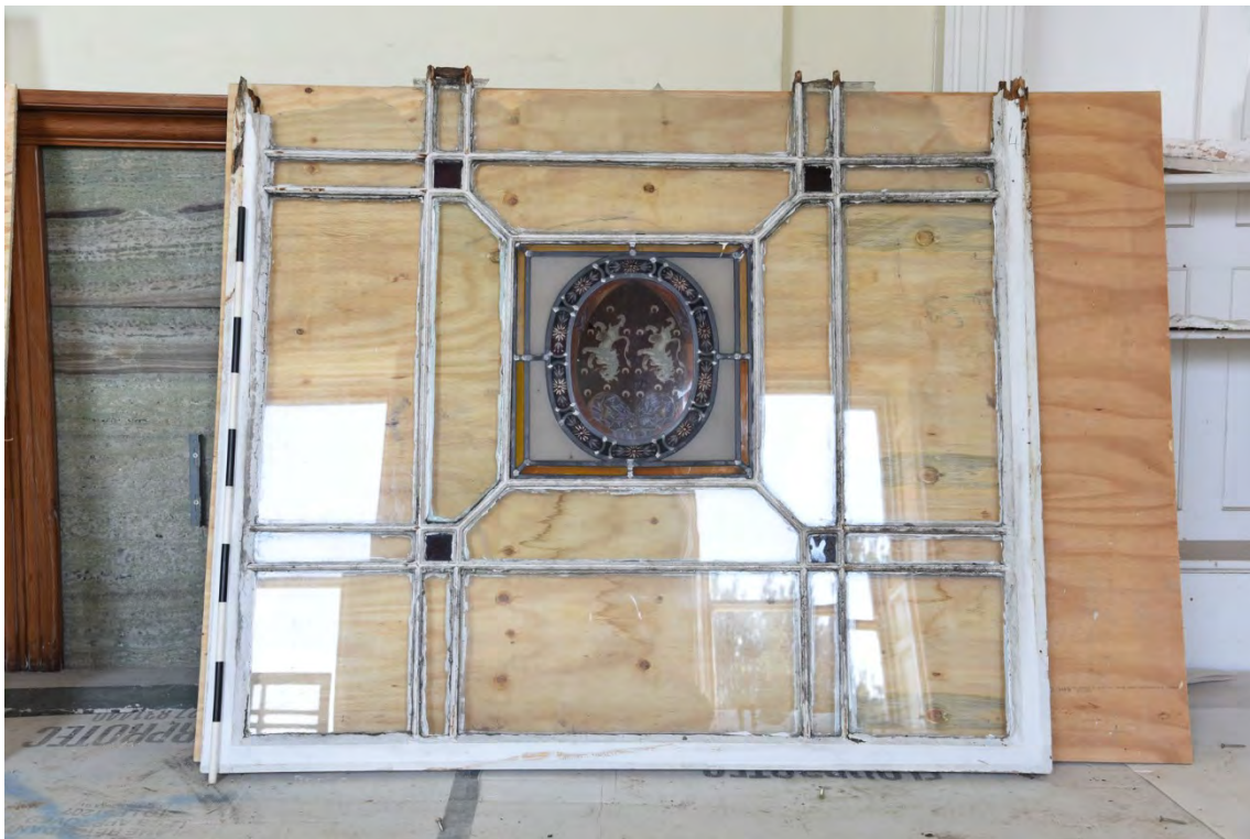
Plate E158 Window panel removed from the lantern's NW elevation, interior view (BRH196)
