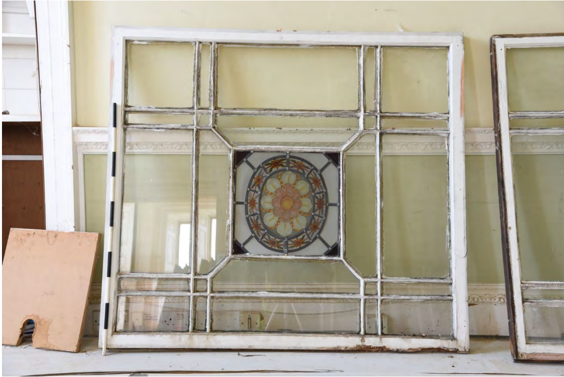
Plate E157 Window panel removed from the lantern's W elevation, interior view (BRH195)
