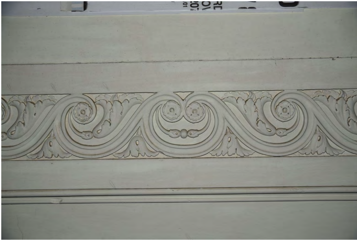
Plate E27 Detail of vestibule decorative plasterwork frieze, looking W (BRH205)
