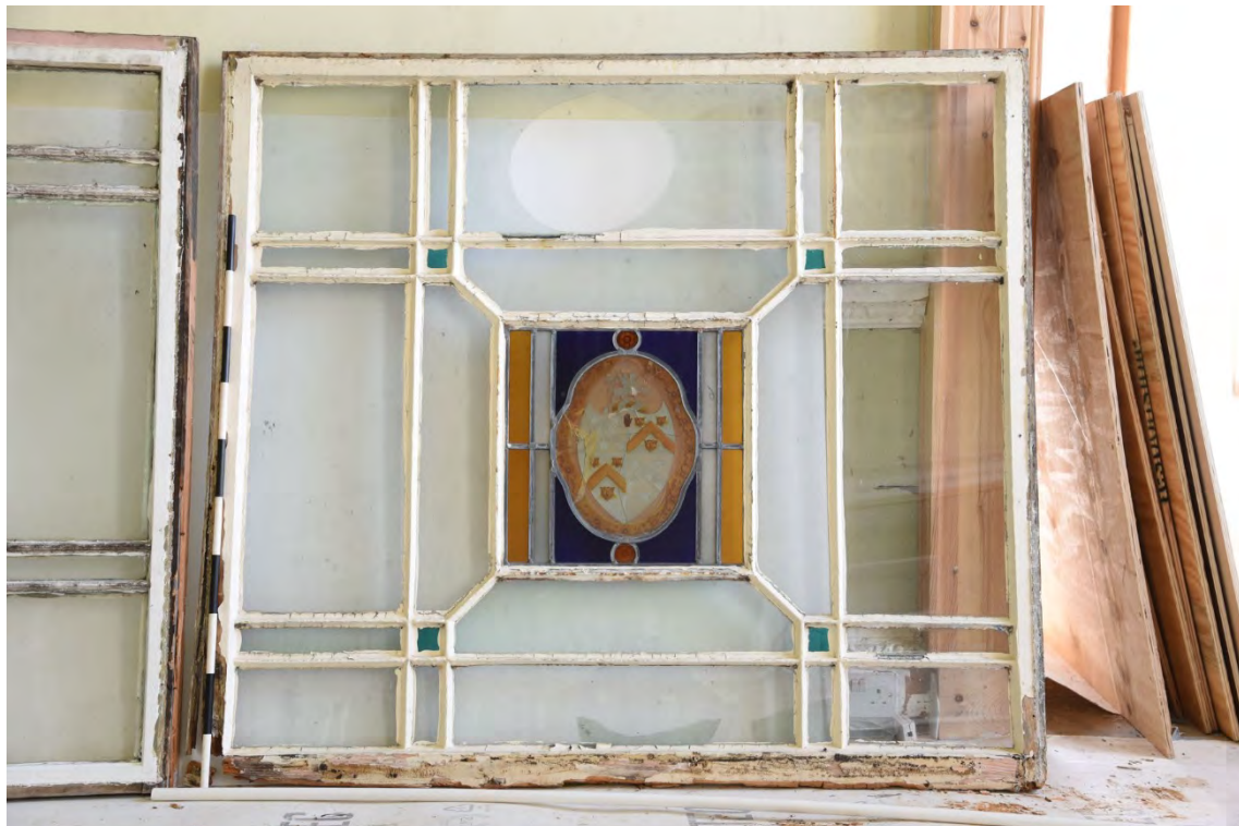
Plate E136 Window panel removed from the lantern's NE elevation, exterior view (BRH172)
