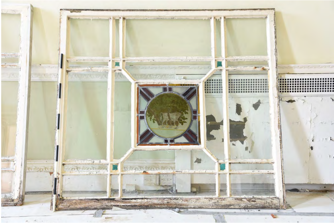
Plate E151 Window panel removed from the lantern's SW elevation, exterior view (BRH189)
