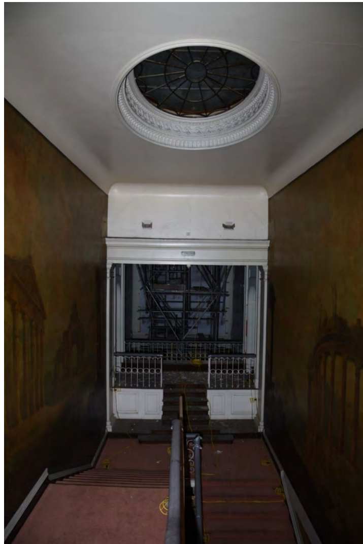
Plate E29 General view into vestibule from staircase at first floor level during works, looking N (BRH207)
