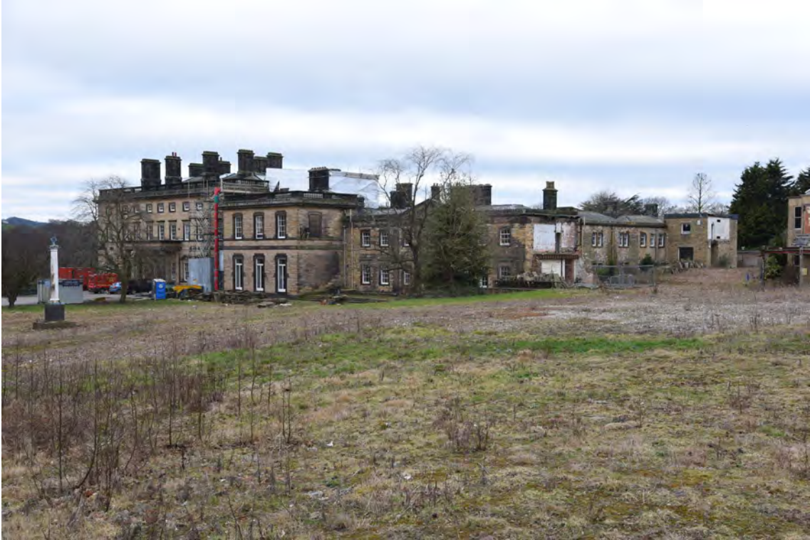
Plate E1 General view of hall looking southwest, showing location of lantern beneath sheeted scaffolding (BRH001)
