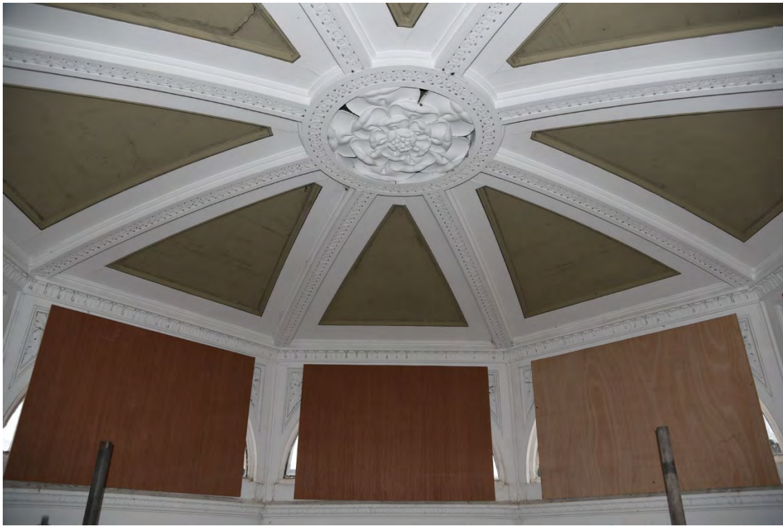
Plate E127 View into the lantern ceiling space looking N, looking N (BRH075)
