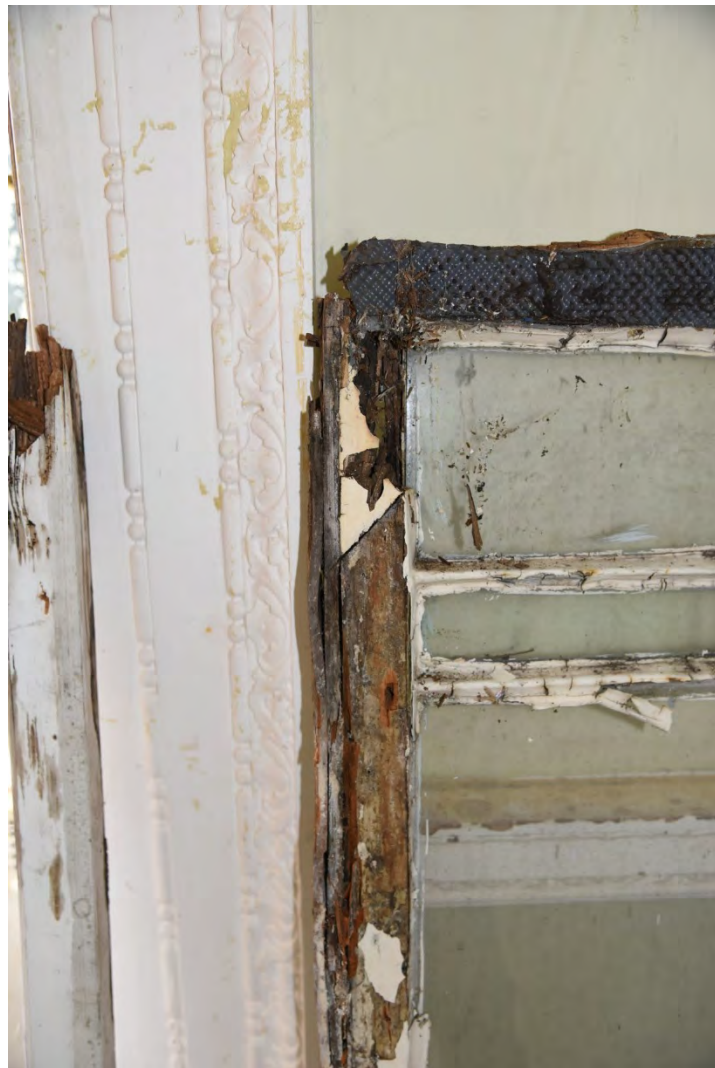
Plate E146 Detail of spliced repair in timber window frame (BRH184)
