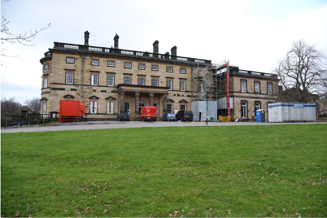
Plate E3 General view of hall looking northwest (BRH003)
