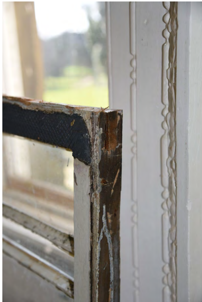
Plate E150 Detail of mortice joint in timber window frame (BRH188)
