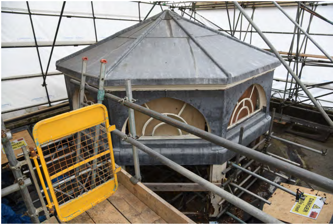
Plate E49 View of lantern roof structure, looking NW (BRH026)
