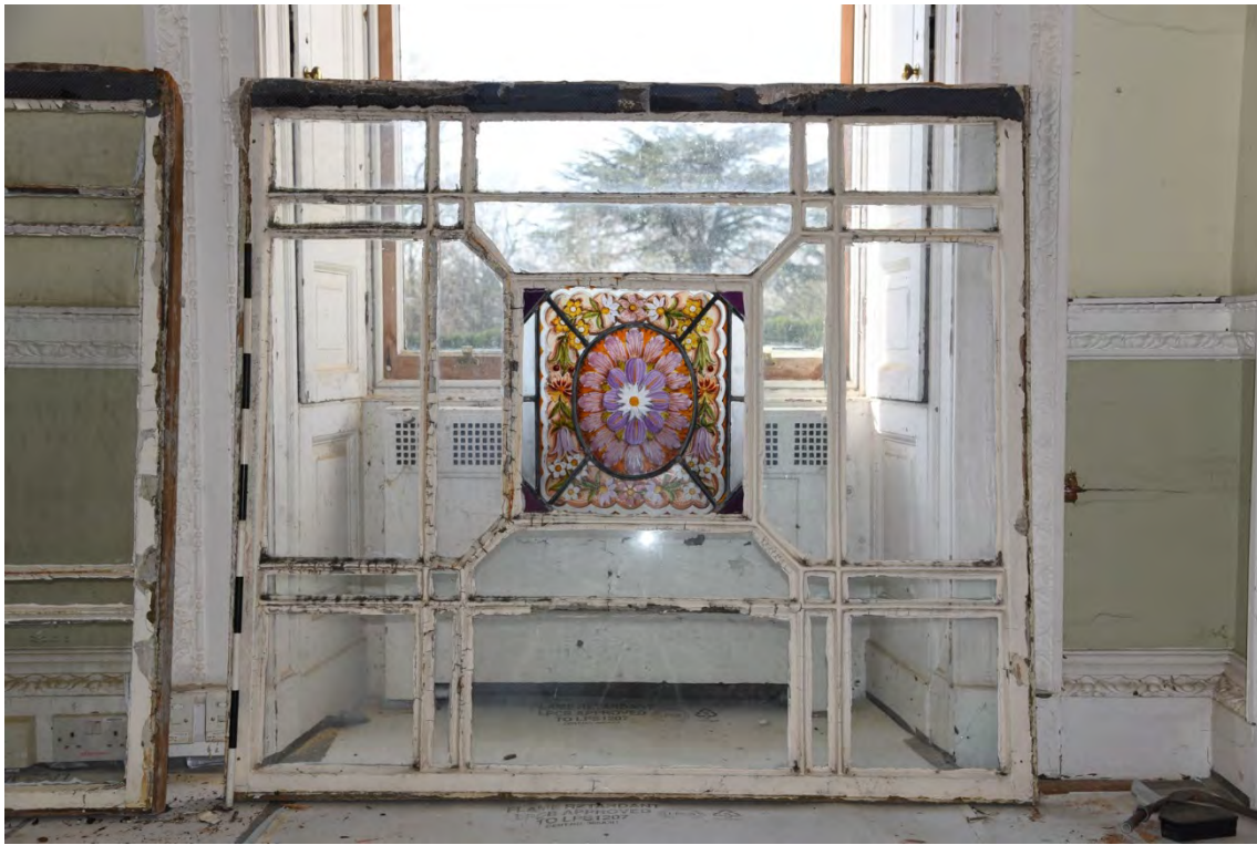
Plate E149 Window panel removed from the lantern's S elevation, exterior view, looking - (BRH187)
