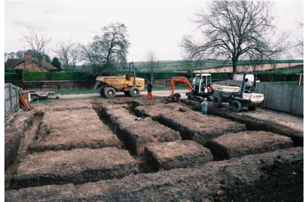
Plate 3 Excavation of footings looking southeast
