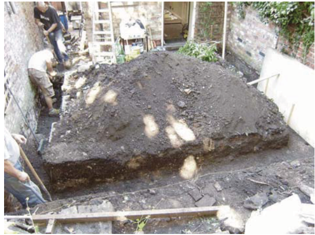
Plate 3 Strip foundations, looking northwest
