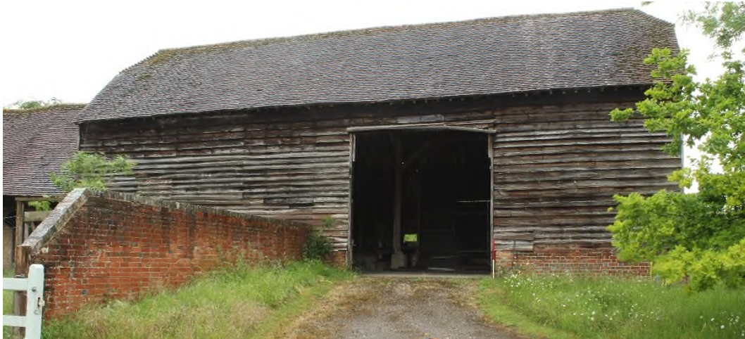
Figure 2 Barn, east elevation.
