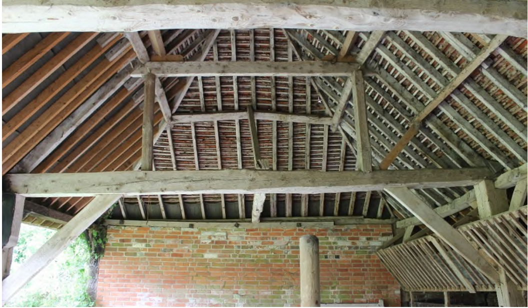
Figure 10 Truss V, north face.
