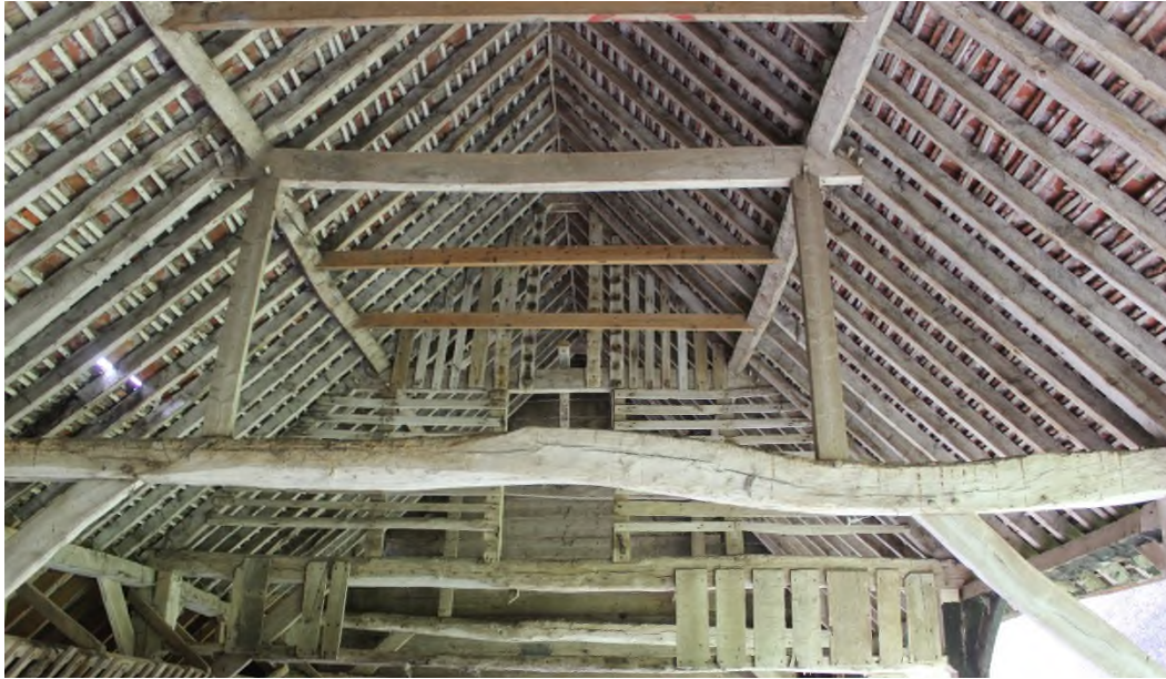
Figure 12 Roof structure looking north with the closed truss, Truss II.
