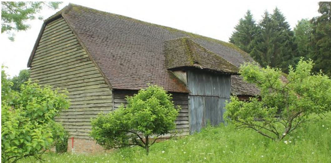
Figure 3 Barn, north and west elevations.
