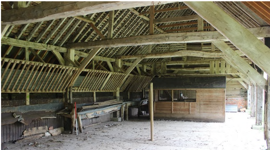
Figure 9 Shelter shed interior facing north-west.
