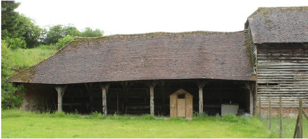
Figure 8 Shelter shed, east elevation.
