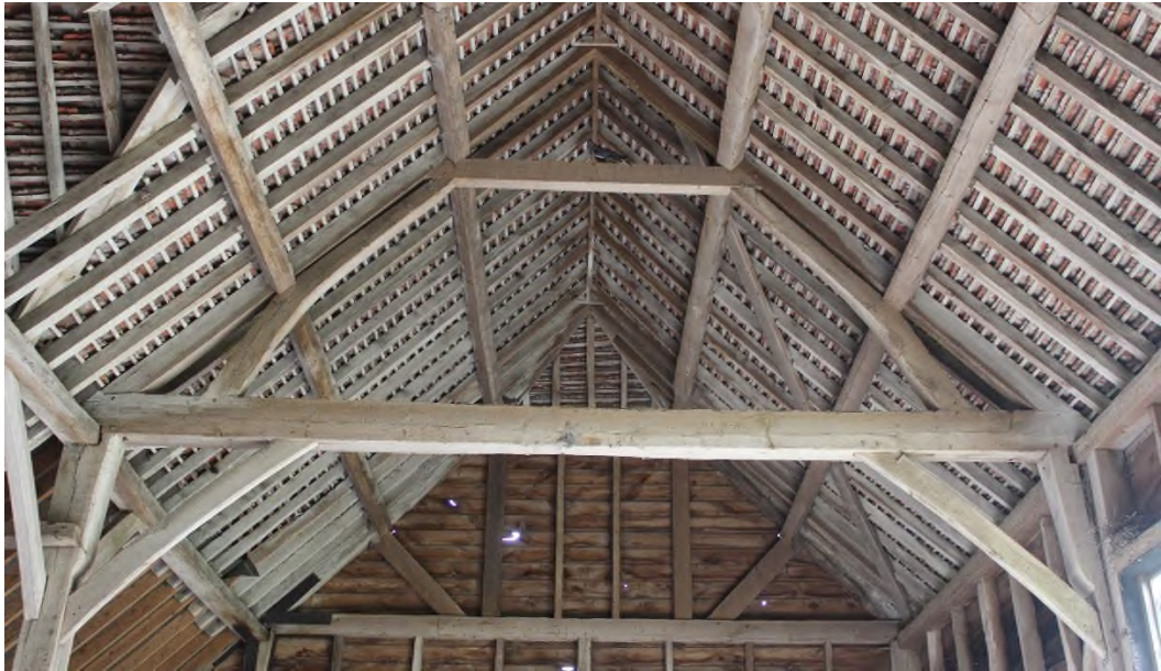
Figure 7 Truss II with inner rafters supporting the lower set of purlins.
