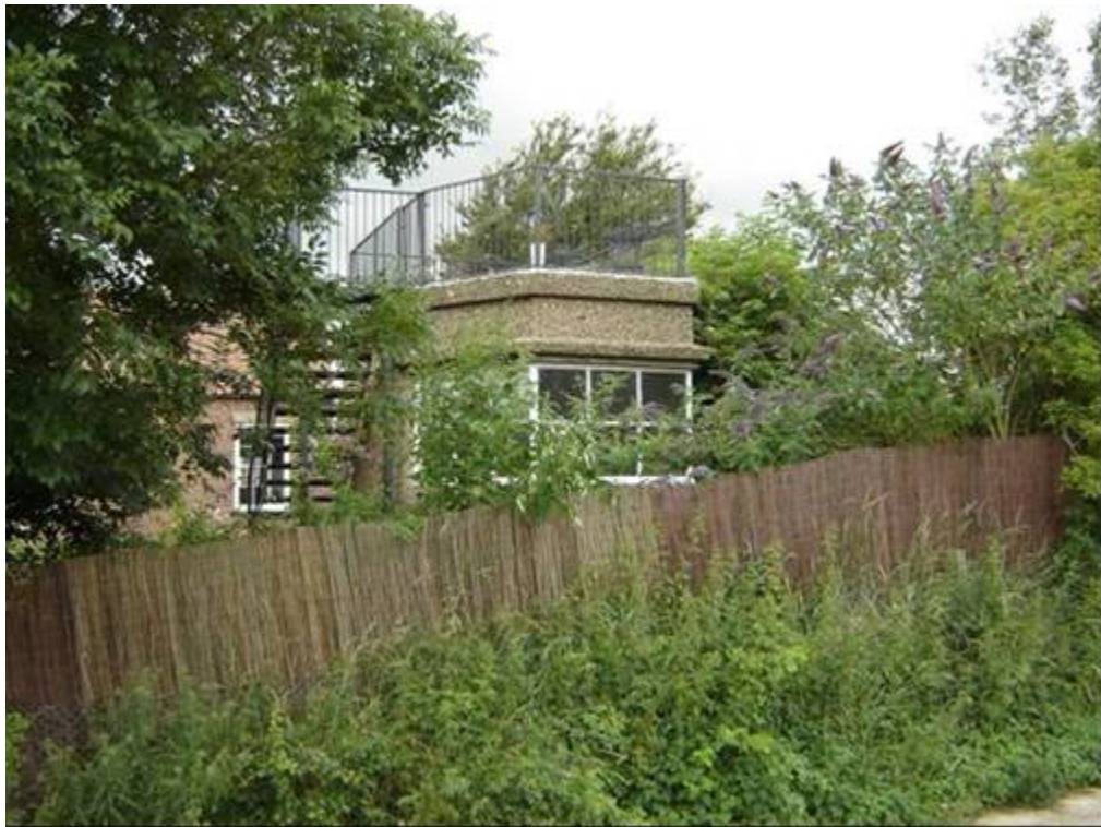
Plate 14 WW2 coast artillery searchlight (CASL) emplacement (FR10) forming part of Freiston Shore Battery, converted to summerhouse on seabank, near TF 3969 4234
