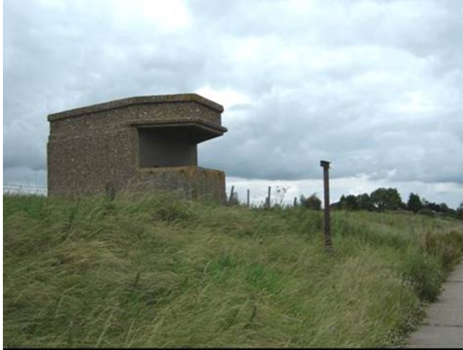
Plate 11 WW2 coast artillery searchlight emplacement (FR20) on seabank forming part of Freiston Shore Battery near TF 3961 4216; this building has been converted to a store by blocking the embrasure and placing a door across the rear access
