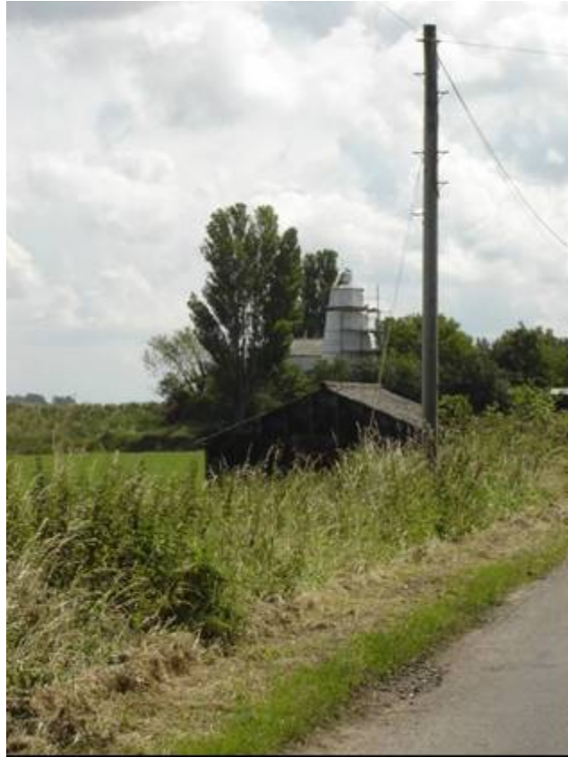
Plate 23 Lighthouse on western side of River Nene, Sutton Bridge (SB5)
