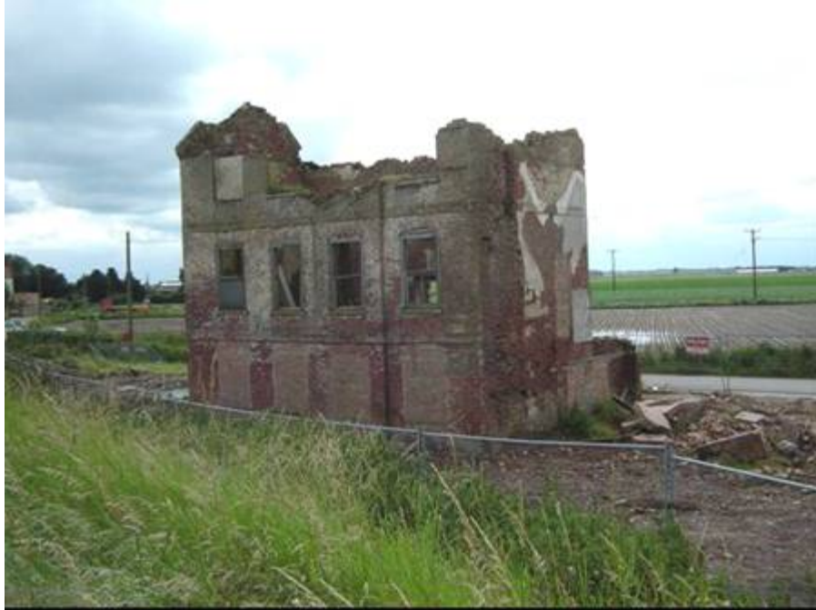
Plate 17 Remains of partially demolished Marine Hotel (FR7), Freiston Shore
