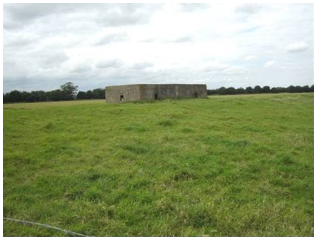
Plate 8 Lincolnshire-type AA pillbox, Butterwick (BU5), taken from south-east
