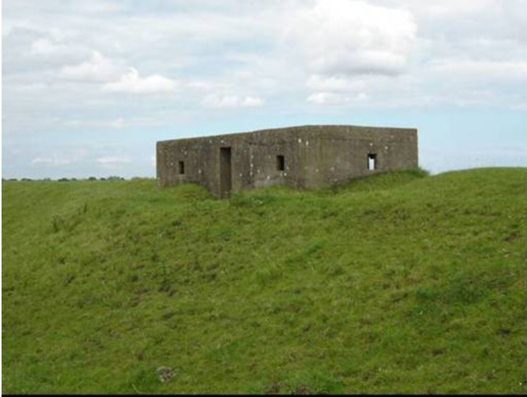
Plate 9 Lincolnshire-type AA pillbox, Butterwick, (BU5) taken from north-west
