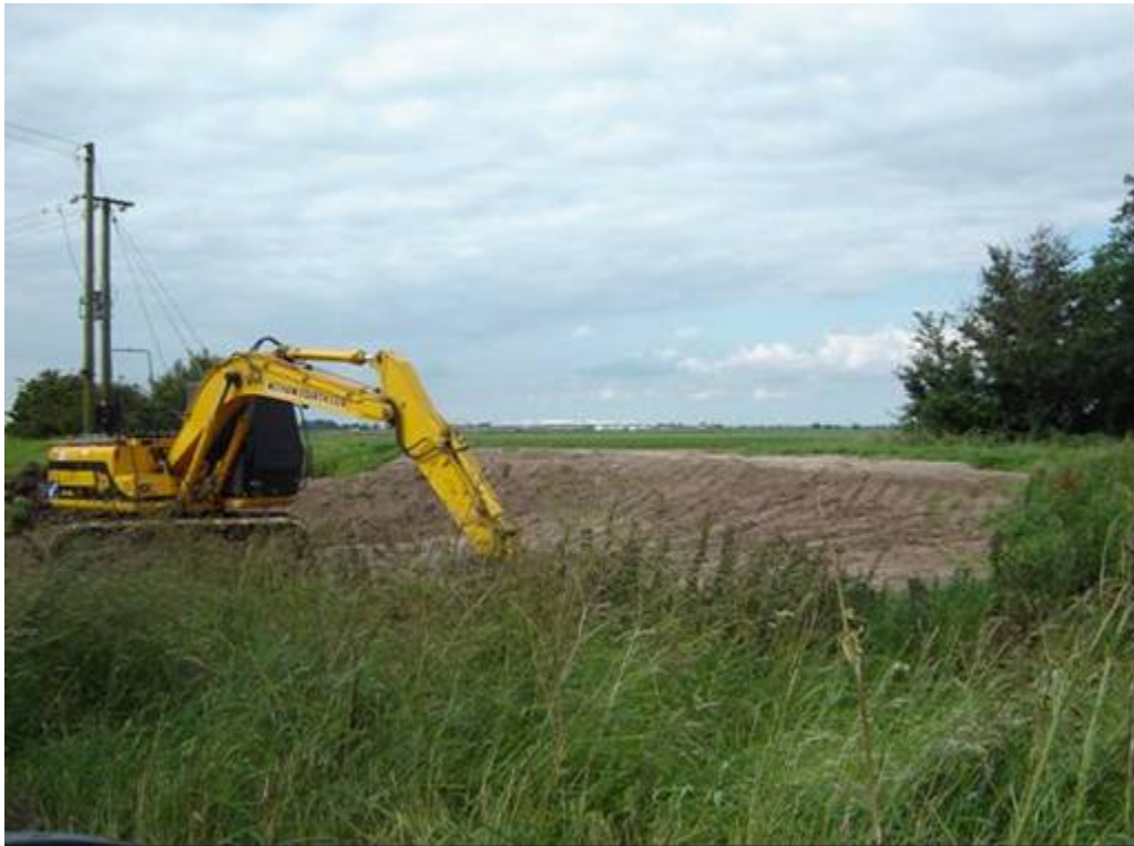
Plate 4 Machine work on north-eastern bank of 'haven' looking north-west (from TF 4329 4948)
