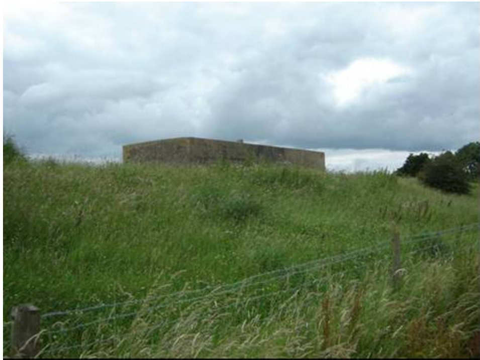
Plate 12 WW2 Lincolnshire-type AA pillbox (FR19) forming part of Freiston Shore Battery near TF 3964 4223
