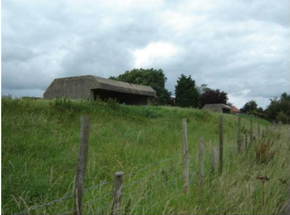
Plate 13 WW2 6-inch gun emplacements (FR9, FR13) on seabank forming part of Freiston Shore Battery near TF 3965 4224
