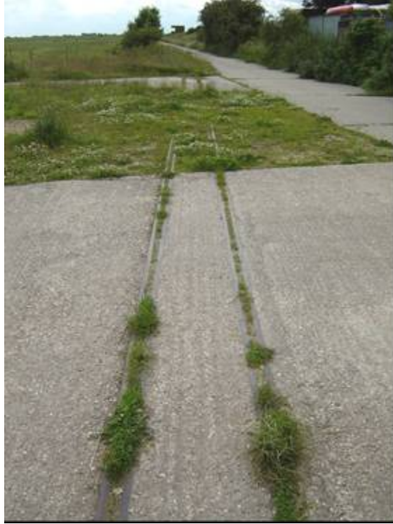
Plate 15 Remains of military railway (FR49), Freiston Shore, at TF 3971 4234
