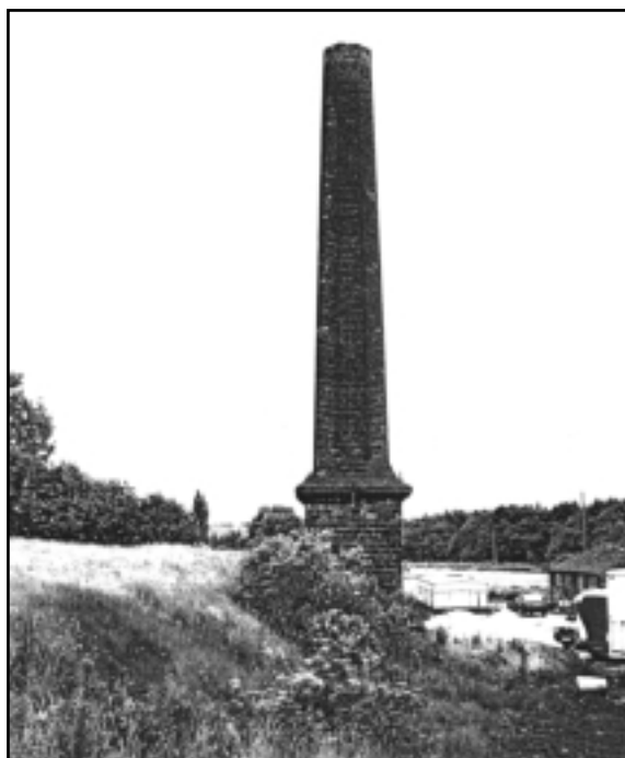
Chimney at the Midland Bleach Works, Cudworth © AS - WYAS
