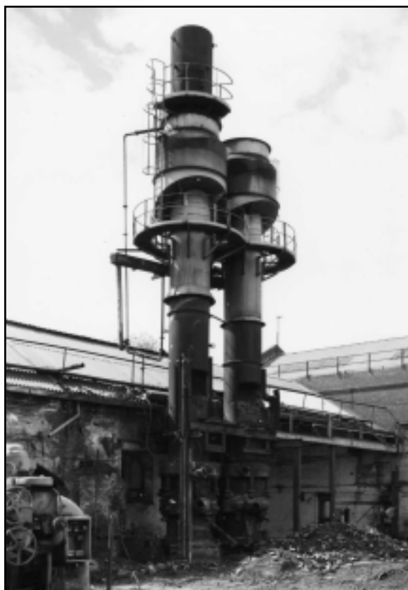
Blast furnace at Vulcan Foundry, Sheffield © AS - WYAS
