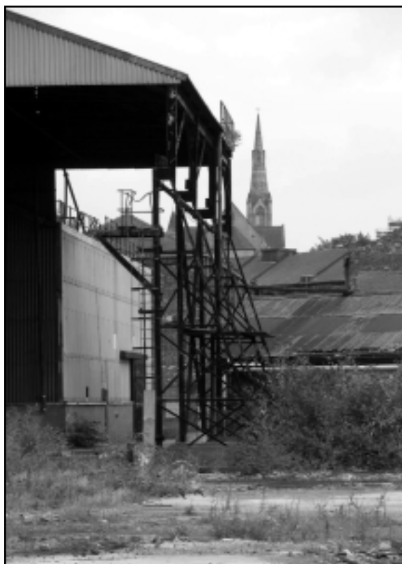
View of foundry building, Guest and Chrimes © SYAS
