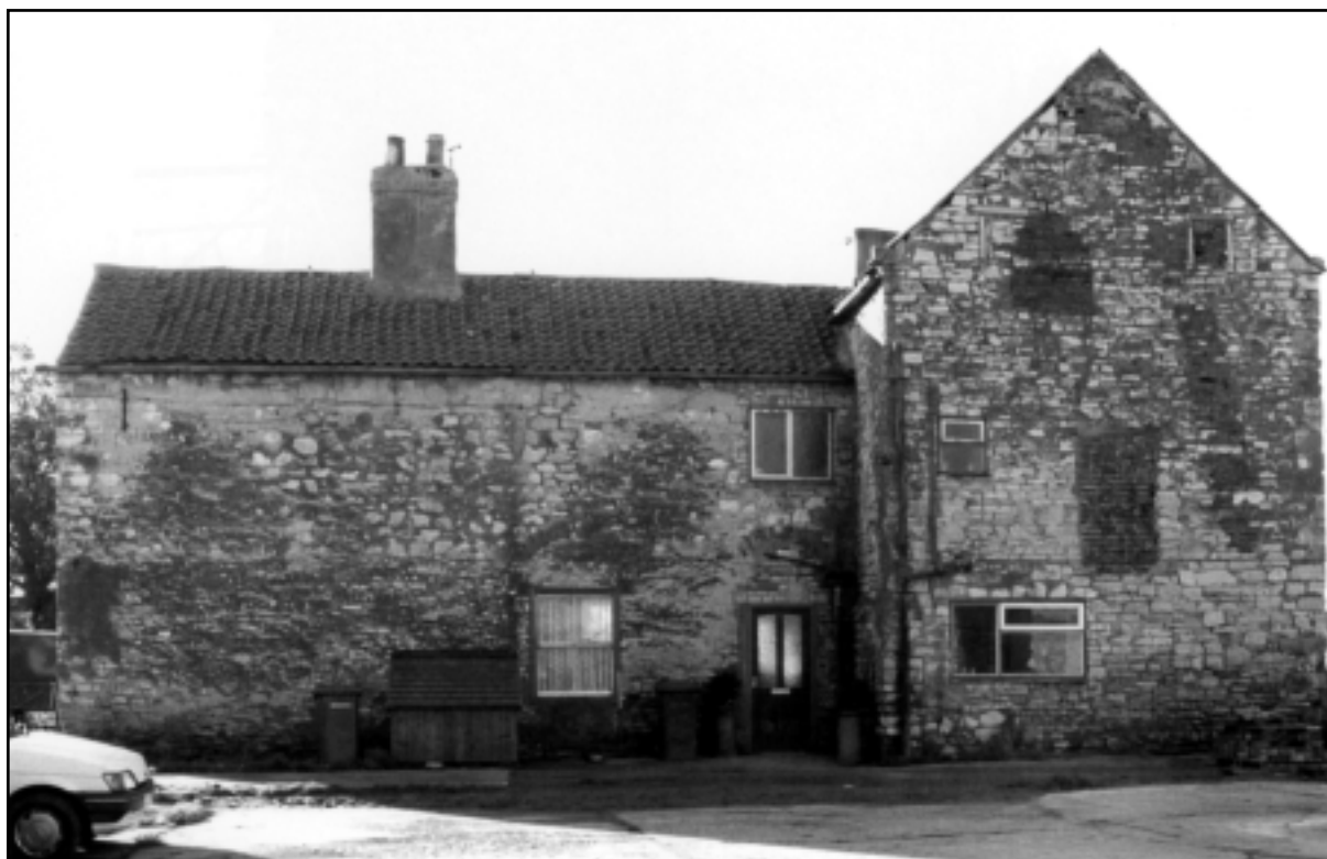
Glebe Farmhouse, Trumfleet. Northern elevation showing blocking in earlier gable © AS - WYAS
