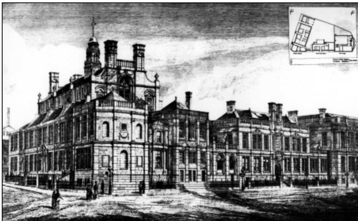
1870s Architects Plan of Firth College, Central Schools and School Board offices, Leopold Street
