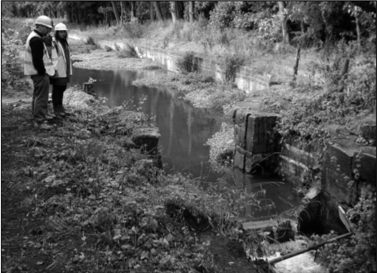
Lock on Chesterfield Canal before restoration © SYAS
