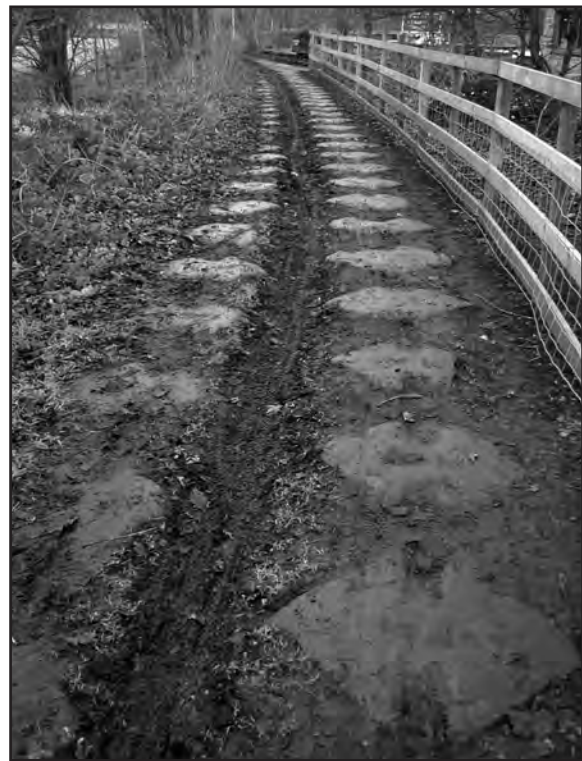
Stone sleepers of Silkstone Railway, built 1809
