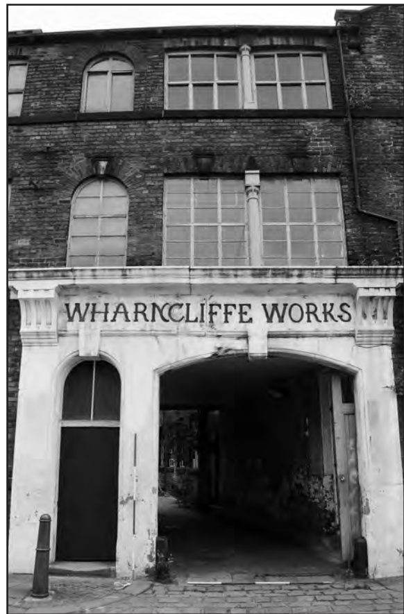
Frontage of the Wharncliffe Works, Sheffield © ARCUS
