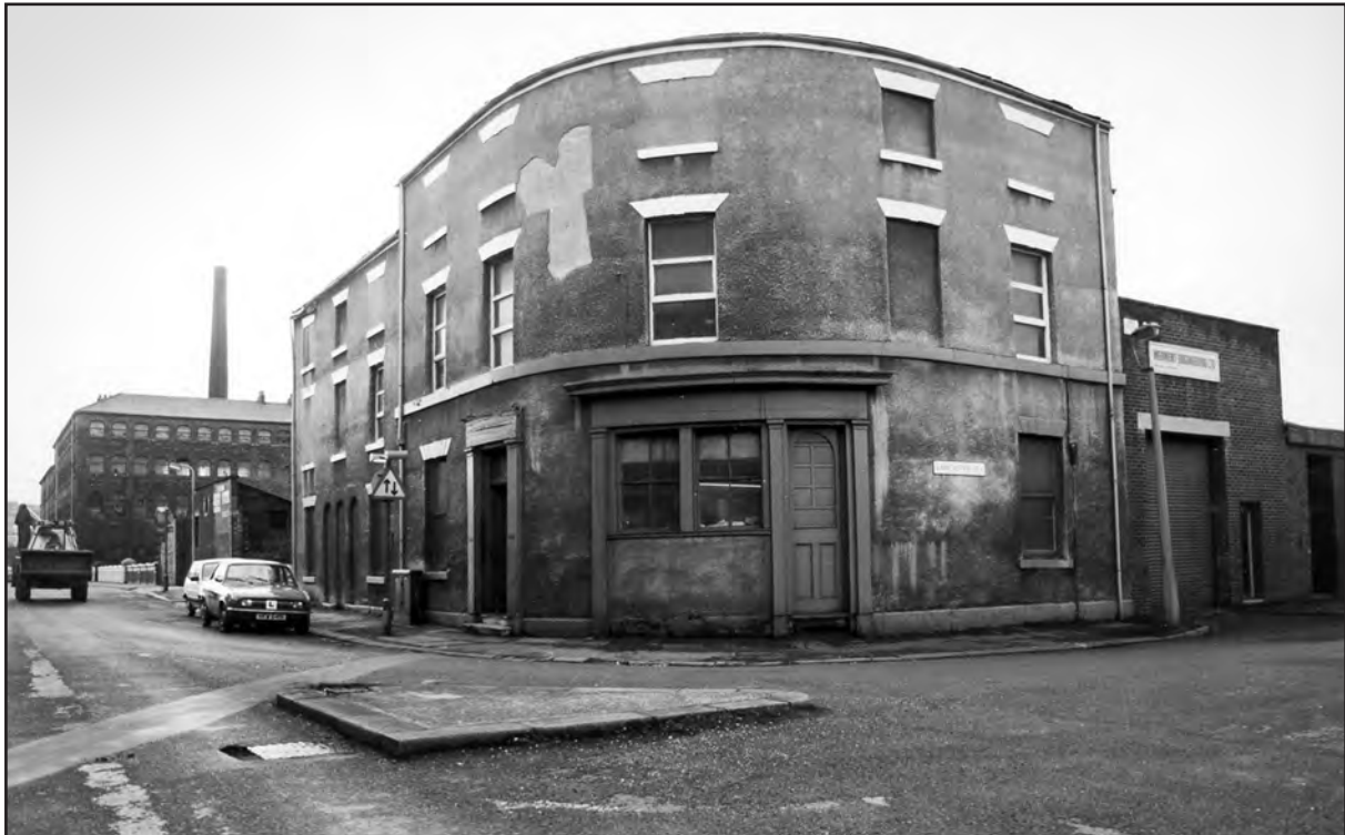
The former Cardigan Tavern at the Lancaster Complex, Ball Street, Sheffield © scc
