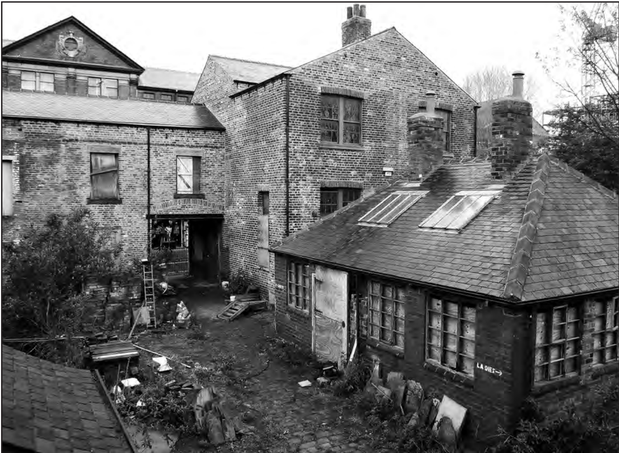
Rear of the Kendal Works, with scissor forge in the foreground © ARCUS
