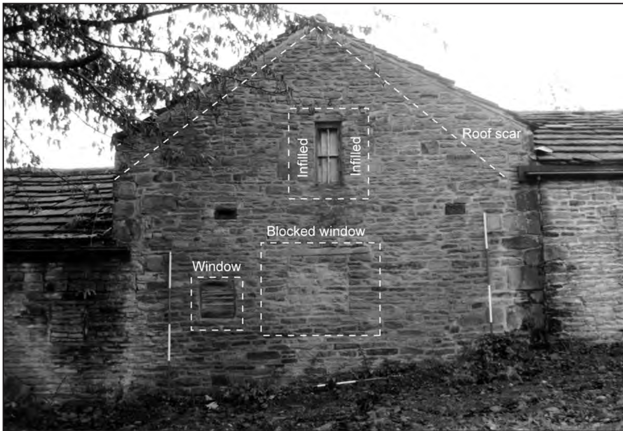
The west gable of the south barn at Abbey Farm © ARCUS
