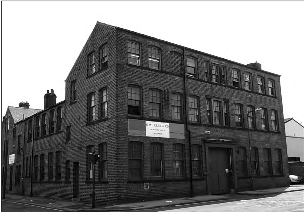
The Murray Building, London Road Student Village © ARCUS
