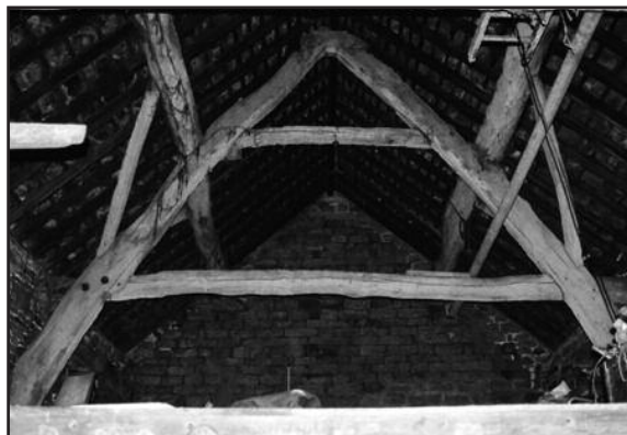
A cruck truss at More Hall Farm, Bolsterstone © ARCUS
