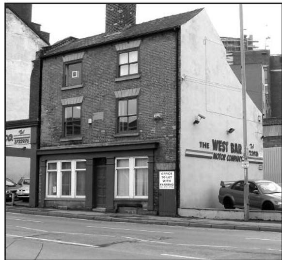
117-119 West Bar, frontage of the listed building with 1794 date stone in the centre © ARCUS
