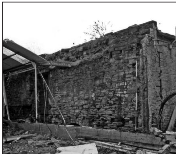
The Don Brewery wall revealed during work at Cornish Square, Sheffield © ARCUS
