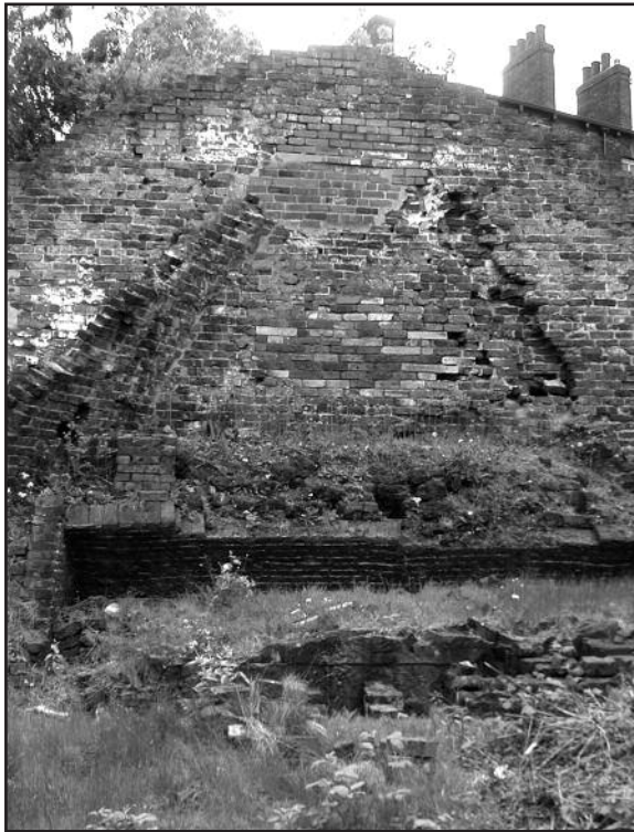
Cementation furnace at Bower Spring, Sheffield, before conservation works © SYAS
