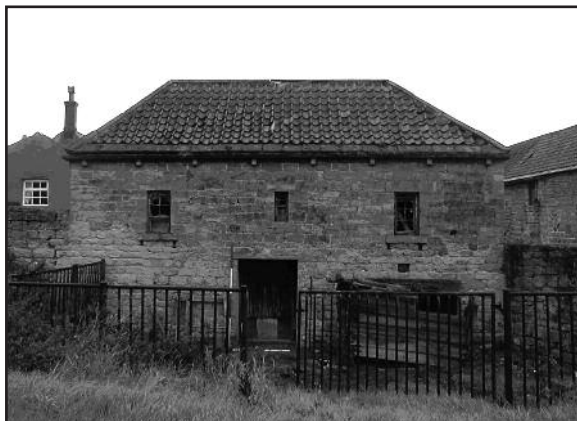
The eastern elevation of the Bull House at Mappleyard Farm © ARCUS
