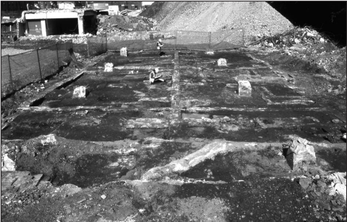
The eastern end of the Union Grinding Wheel under excavation © ARCUS
