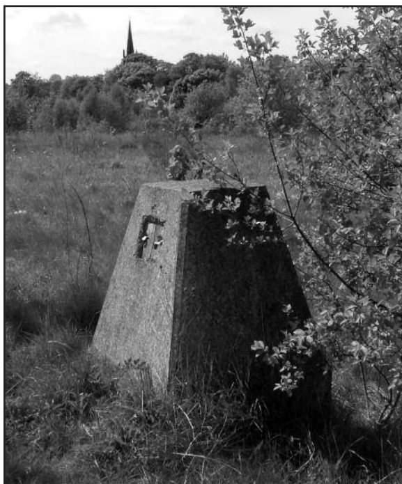
Concrete cap marking the location of a shaft, Elsecar Main Colliery © ARCUS
