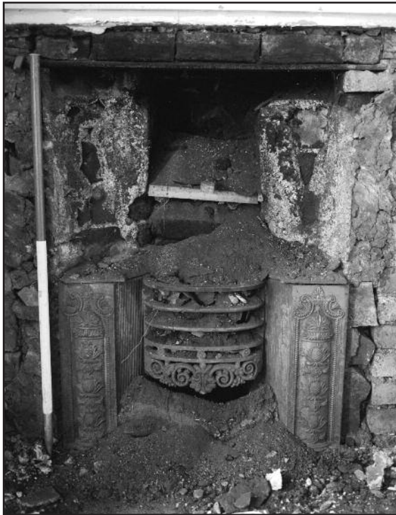
A fireplace with cast iron grate in the east range of Leah's Yard, Cambridge Street
