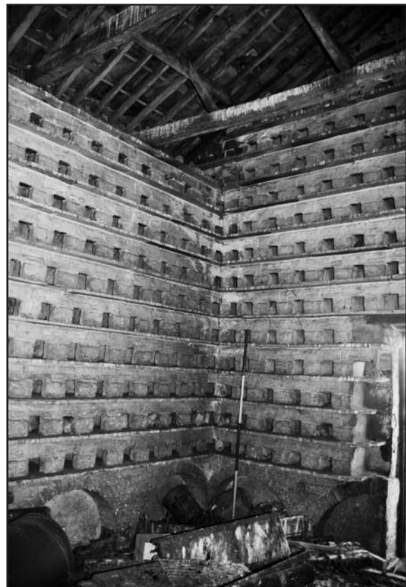
Detail shot showing dove nest-boxes in the dovecote at Low Laithes Farm © CS Archaeology
