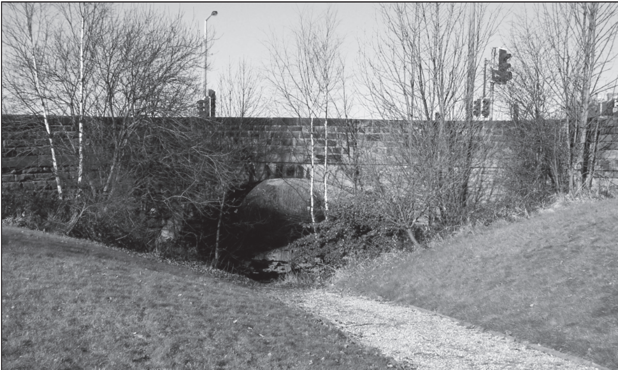
The nineteenth century coal railway tunnel at the junction of Old Mill Lane and Burton Road © ARCUS
