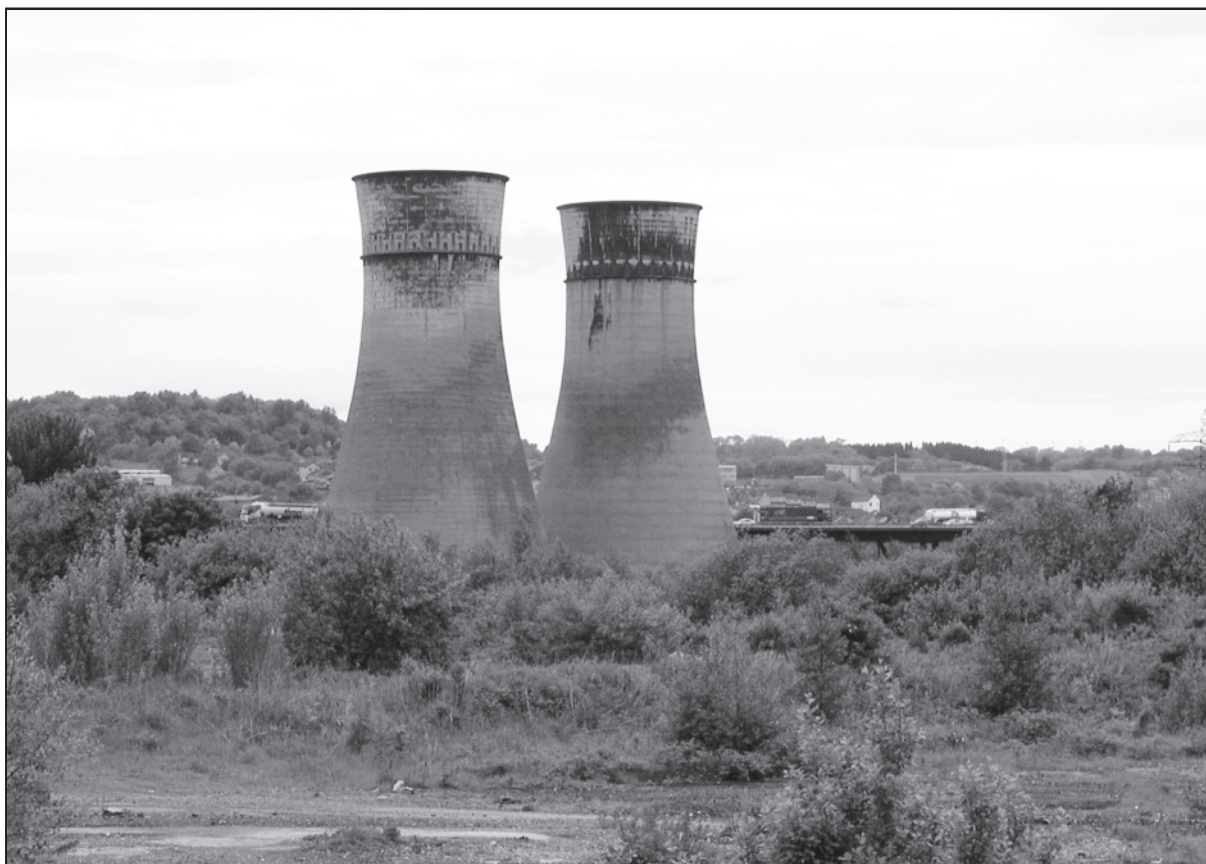
Tinsley Cooling Towers, remains of the Blackburn Meadows power station © SYAS
