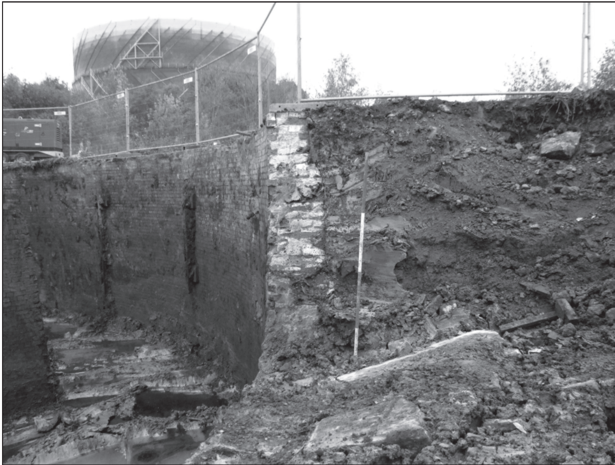
Section through former gasholder, Old Mill Gas Works © ARCUS
