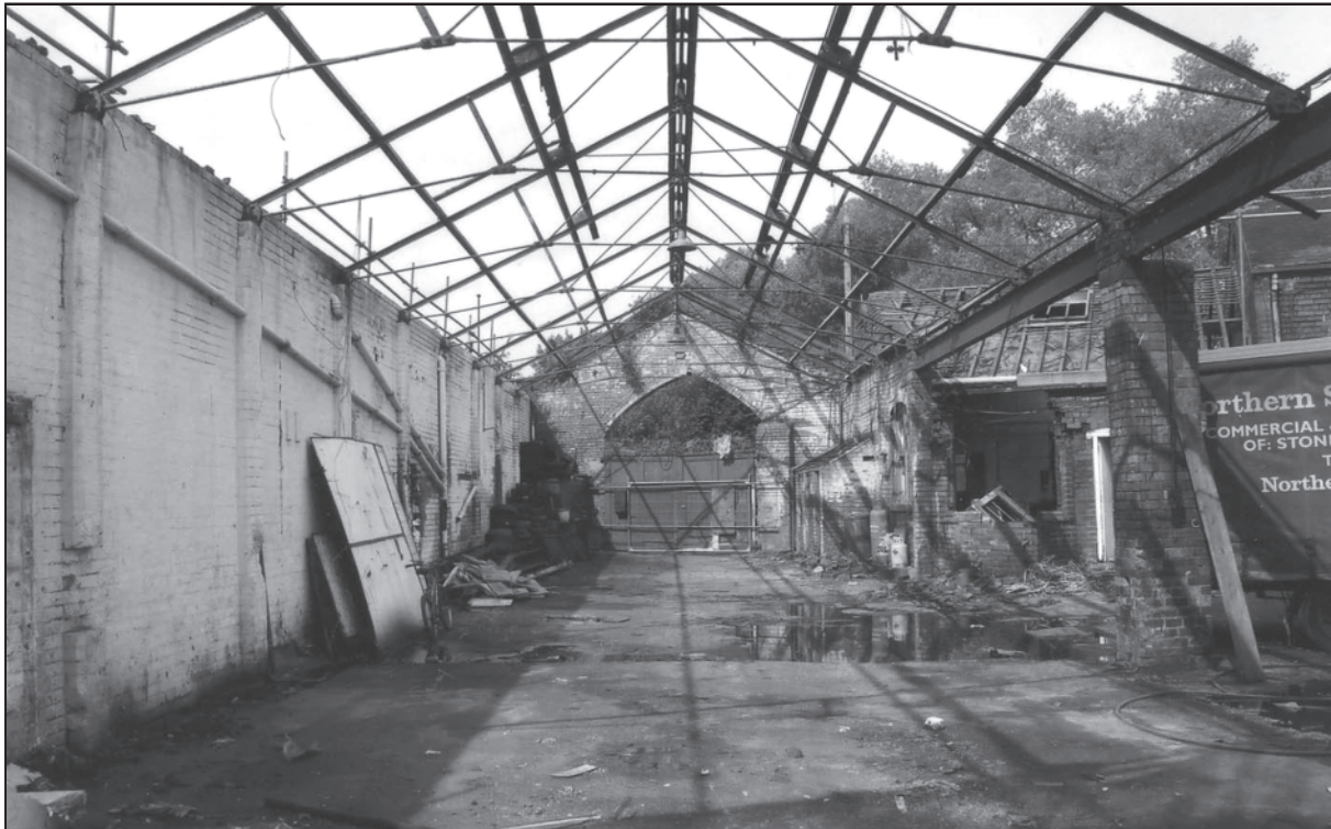
Internal view of former tram shed, Albert Road, Heeley © ARCUS
