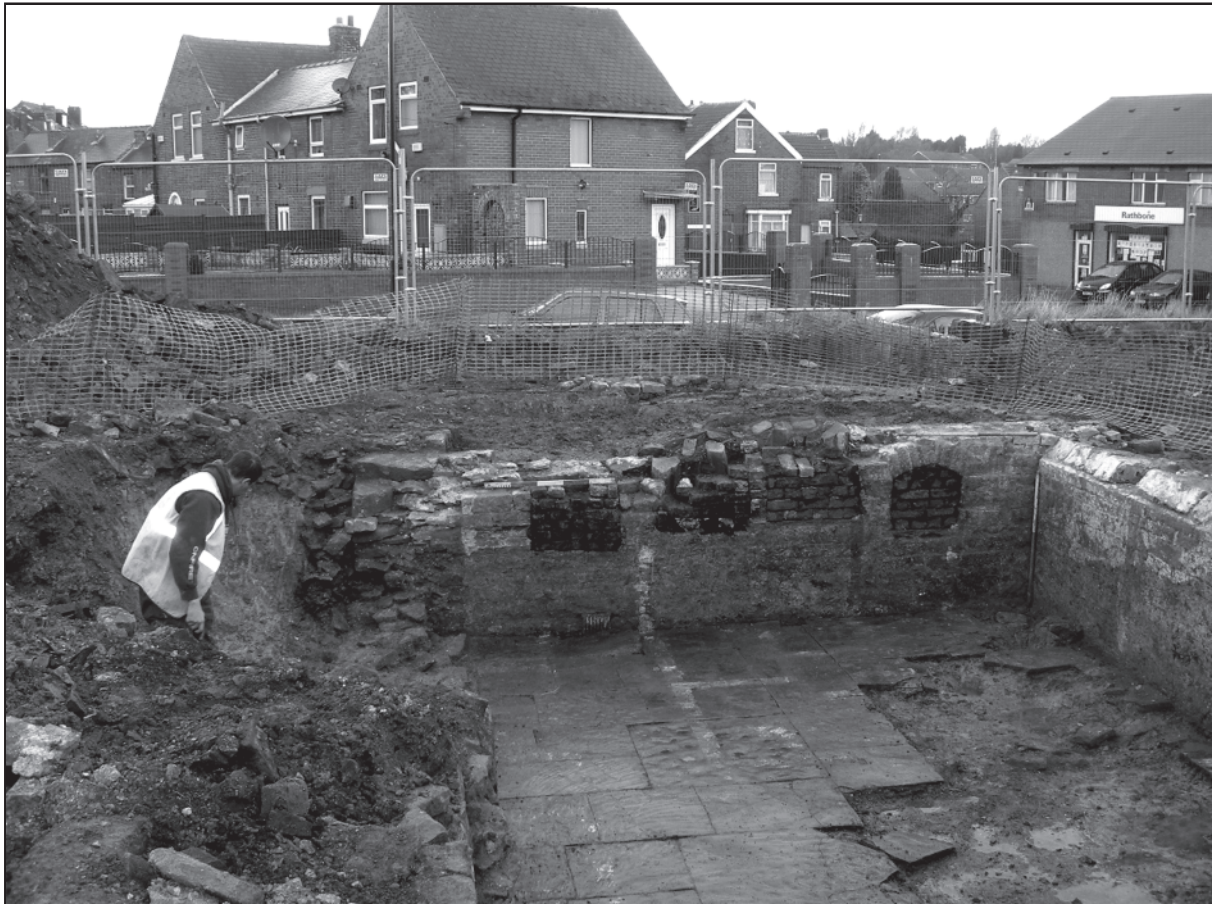
Remains of cellar from Wincobank Hall showing blocked lightwell and alcoves © SYAS
