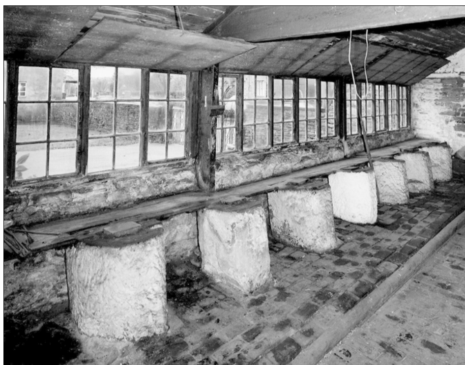
Figure 3 Interior of file cutters' workshop, Crown File Works, 11 High Street, Ecclesfield (NMR: AA98/14082). Crown File Works is a complex of sandstone buildings built around a smallholding, dating from the early 19 th century. It is a good surviving example of a combined agricultural and industrial complex comprising a farmhouse, stable, file cutters' workshop, packing shop, hardening shop, tanging shop and forge, and cartshed (© English Heritage)
