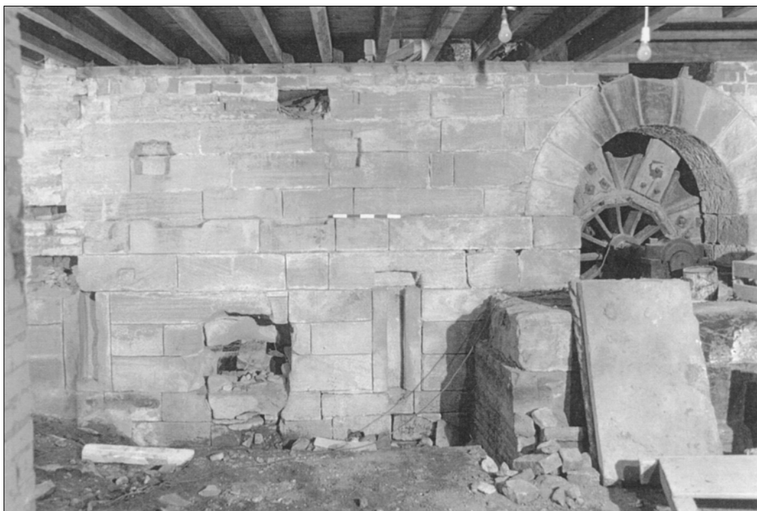
Figure 24 Gearing wall inside building 1 at the Saw Mill, showing location of phase 2 hursting (© Archaeological Services, WYAS)
