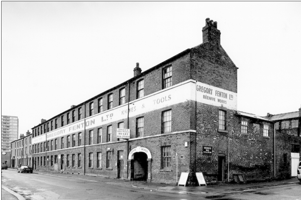
Figure 2 Beehive Works, Milton Street, Sheffield (NMR: AA98/13962). Beehive Works, originally known as Milton Works, is a large complex, arranged around two courtyards, which manufactured cutlery, silver plate and files. All the main buildings on the site were built between the 1860s and 1890. It has a front range, containing offices, showrooms and a warehouse, with workshop ranges round the courtyards, containing forges, grinding hulls and cutlers' workshops (© English Heritage)
