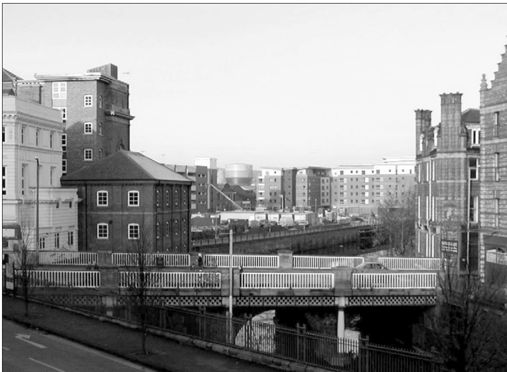
Figure 5 Lady's Bridge on the River Don (© SYAS)
