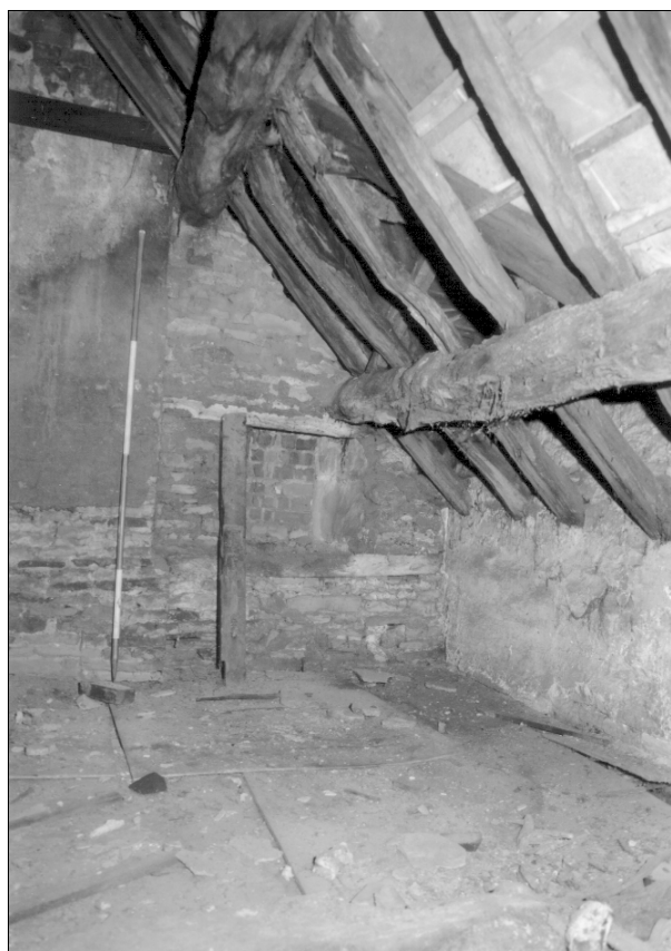
Figure 22 Barugh Lane Farm, showing blocked window in gable, and ridge of barn running into the upper purlin of the house (© Archaeological Services, WYAS)
