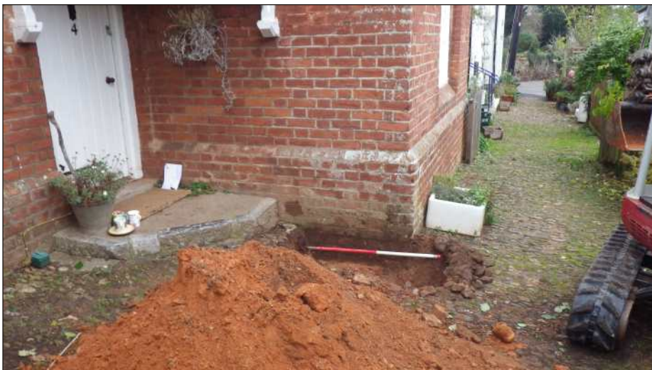
Plate 3: Geotechnical Test Pit 3, looking east (scale 1m)
