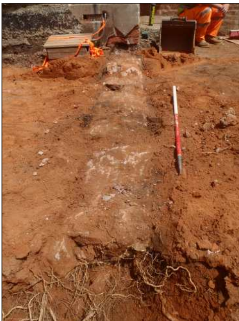
Plate 7: Site-wide levelling, garden wall foundation F0026, looking east (scale 1m)
