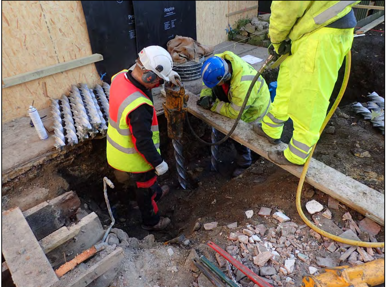
Plate 5: Driving 'Heli' piles into base of foundation trench
