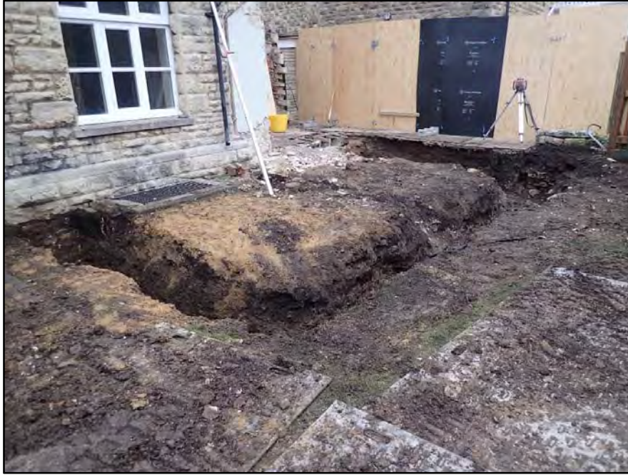
Plate 1: Overview of excavated foundation trench, viewed from S
