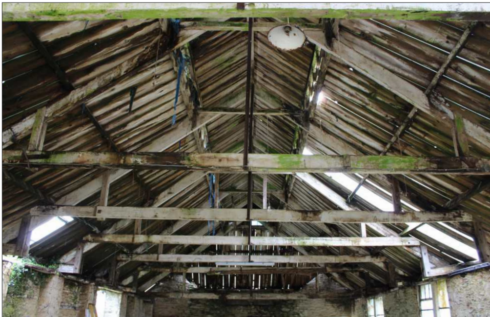
Plate 12: Roof structure, looking northeast
