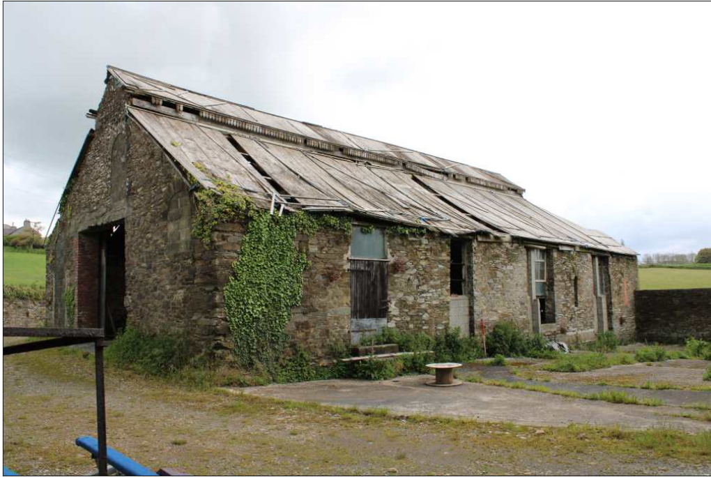
Plate 5: Southeast elevation, looking north-northeast (1m scale)
