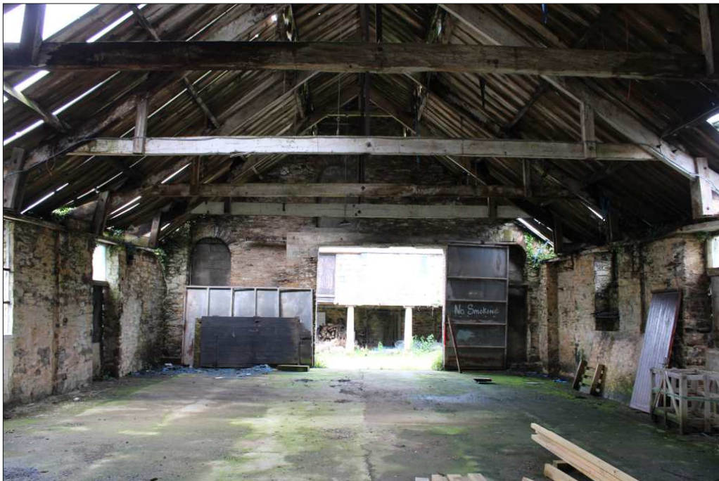
Plate 8: Internal view of the barn, looking southwest (1m scale)
