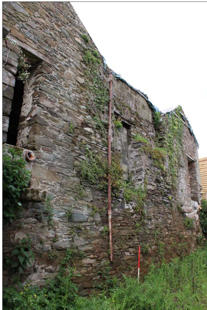
Plate 2: Northeast elevation, looking northwest (1m scale)
