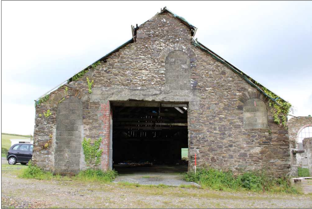
Plate 7: Southwest elevation, looking northeast (1m scale)
