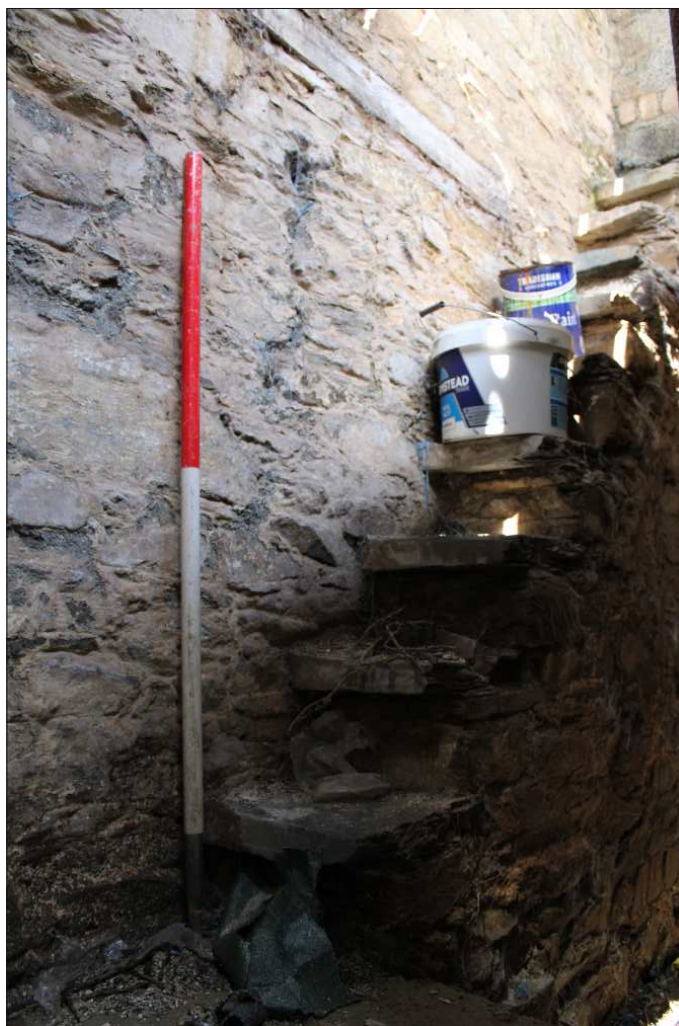
Plate 13: Stone steps on the southwest wall, looking northwest (1m scale)
