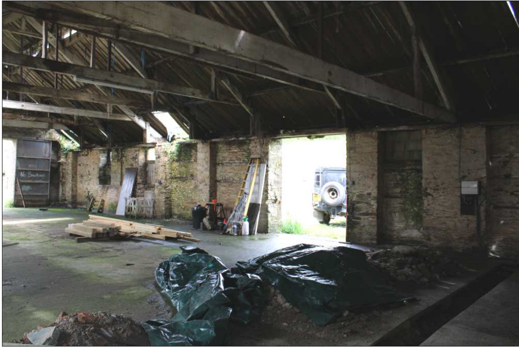
Plate 11: Internal view of northeast wall, looking northwest (1m scale)
