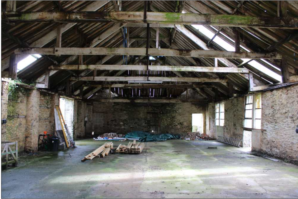
Plate 9: Internal view of the barn, looking northeast (1m scale)
