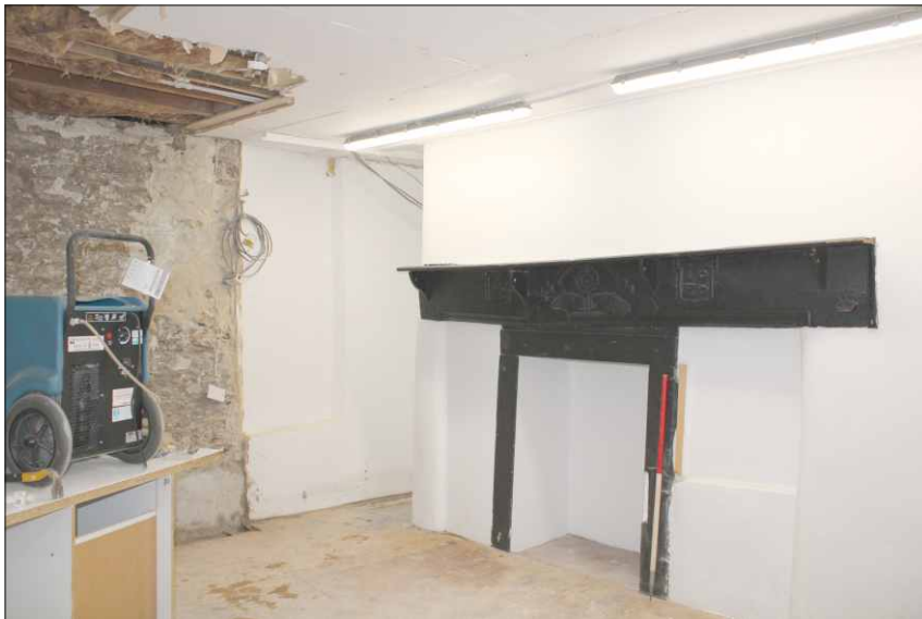
Plate 2: View of the fireplace within the room, looking north-northwest (1m scale)
