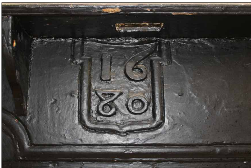
Plate 6: Detail of the right carving on the fireplace, looking north-northeast
