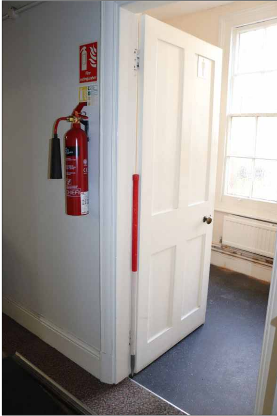
Plate 10: 19th-century four-panel door in staff welfare block, looking north (1m scale)
