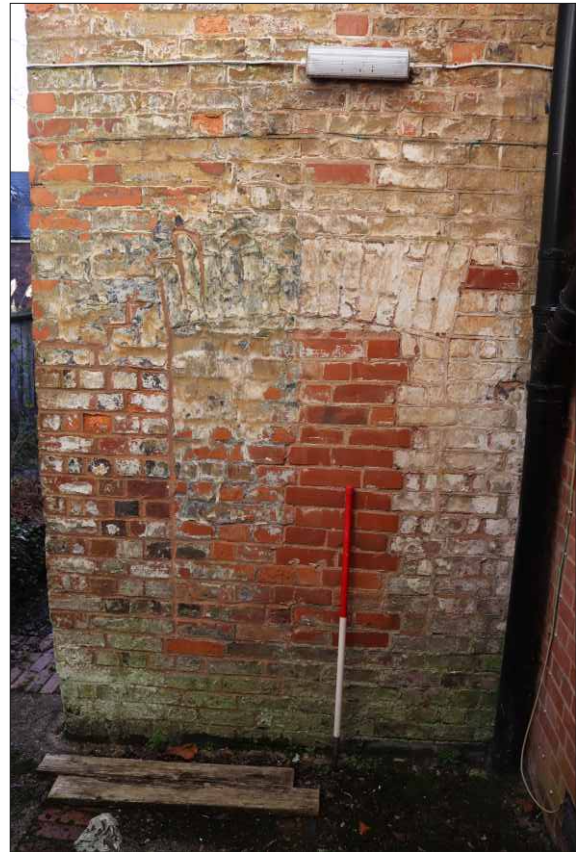
Plate 6: North elevation of the staff welfare block, looking southeast (1m scale)
