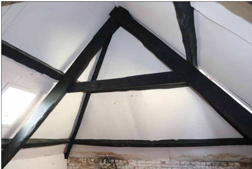
Plate 23: Roof truss in No. 31, looking west
