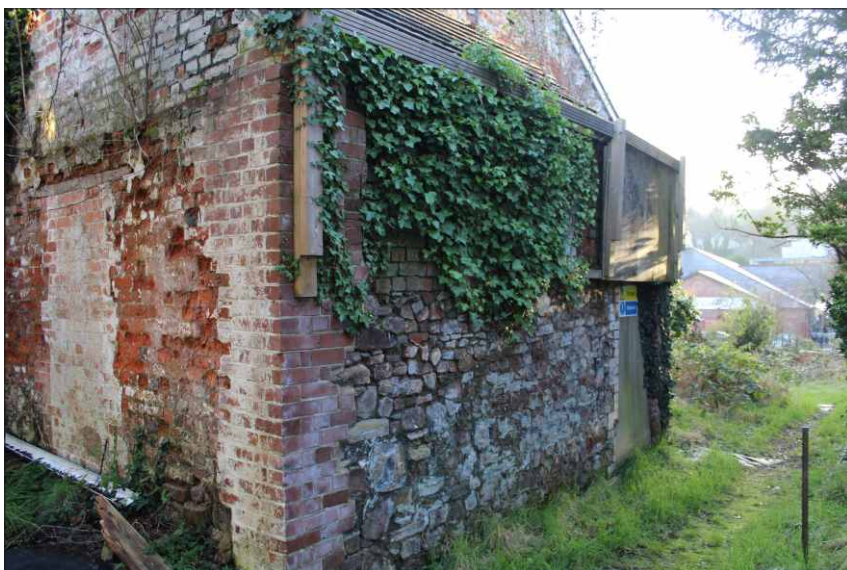
Plate 24: Outbuilding, looking east
