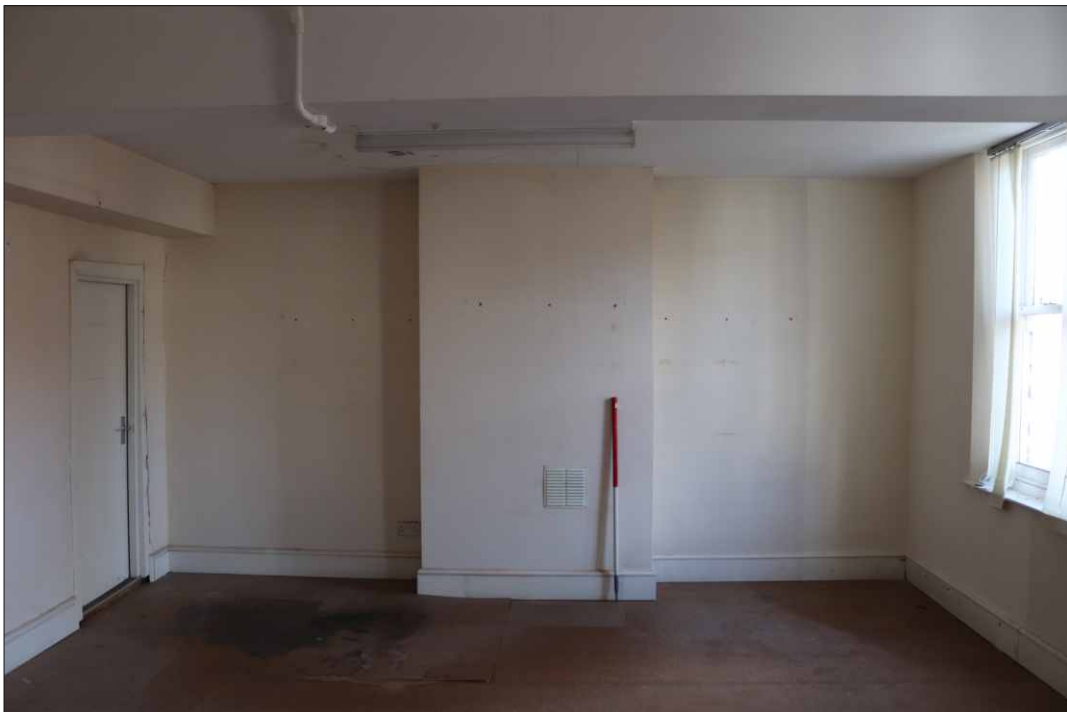
Plate 17: Second floor front room (201) in No. 29, looking southwest (1m scale)
