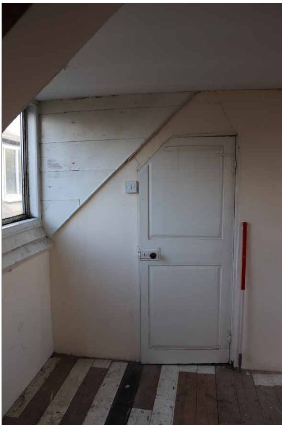
Plate 20: 18th-century door on third floor of No. 29, looking southeast (1m scale)
