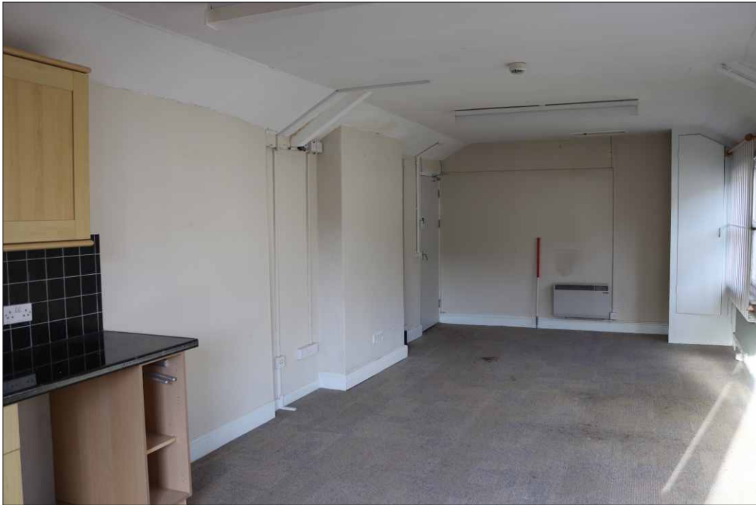
Plate 16: First floor room of staff welfare block, looking northwest (1m scale)
