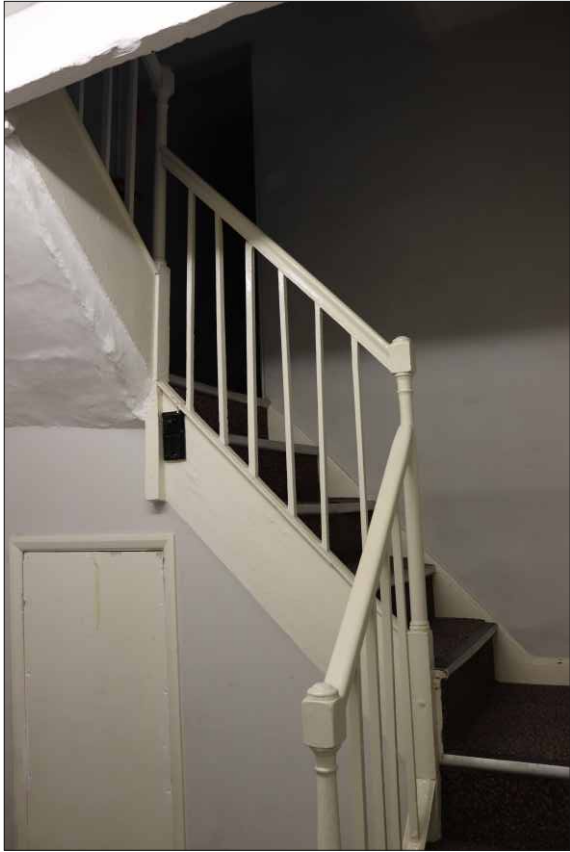
Plate 13: Stairs from first to second floor in No. 29, looking south
