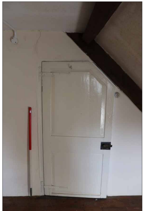
Plate 21: 18th-century door on third floor of No. 29, looking northwest (1m scale)
