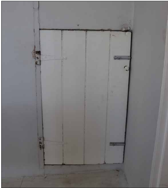
Plate 22: 19th-century door on third floor of No. 29, looking northwest
