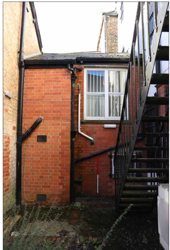
Plate 4: East elevation of link structure, looking southwest (1m scale)
