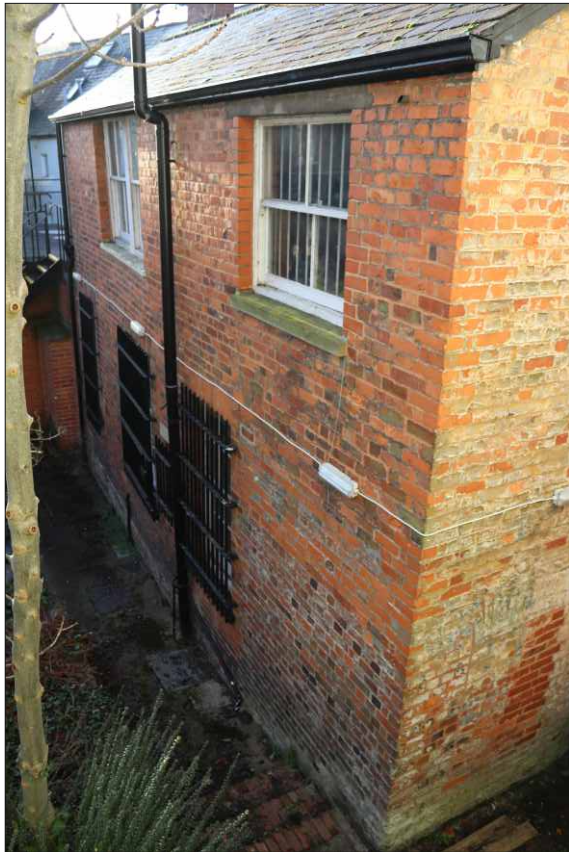
Plate 5: East elevation of the staff welfare block, looking south
