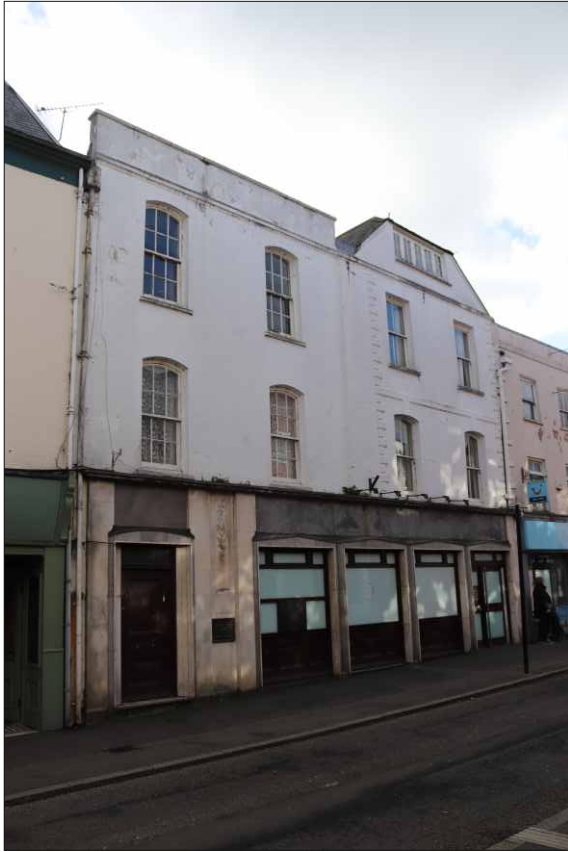
Plate 1: Main façade on Fore Street, looking southwest
