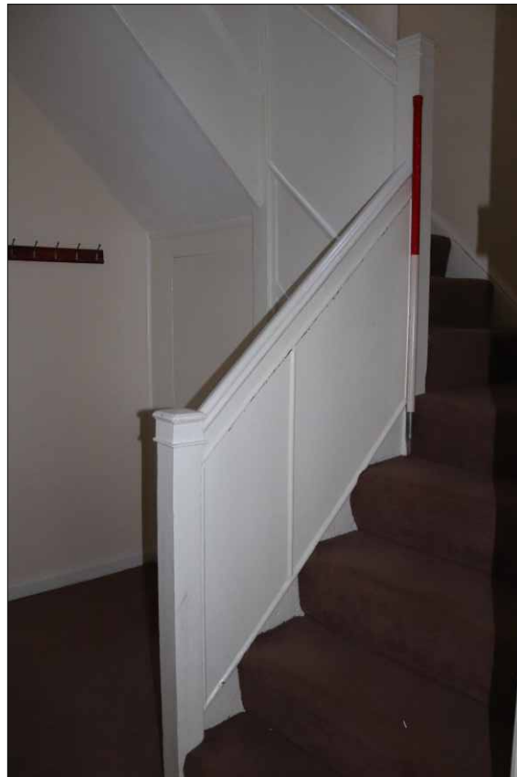
Plate 15: Stairs from first to second floor in No. 31, looking north (1m scale)
