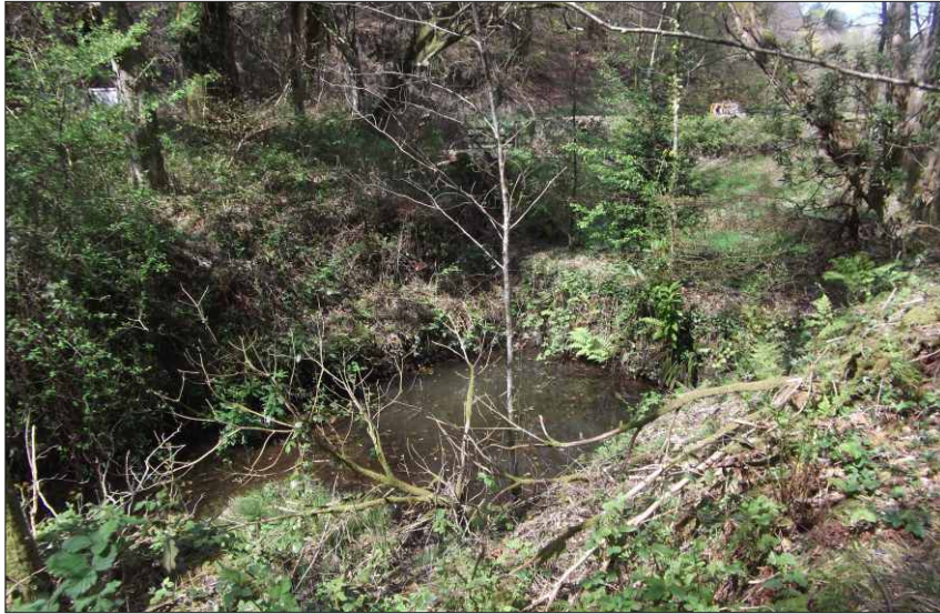
Plate 1: Boathouse or docking bay, Old Brockham Bridge, looking northwest
