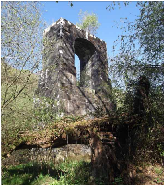
Plate 2: East bridge pier, looking northwest
