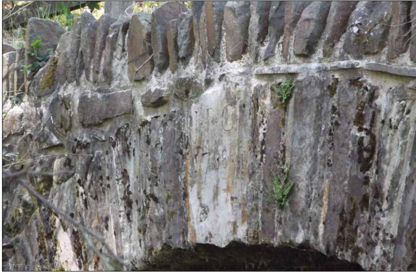
Plate 4: Smallacombe Bridge, date on keystone 'JPC 1788', looking northwest
