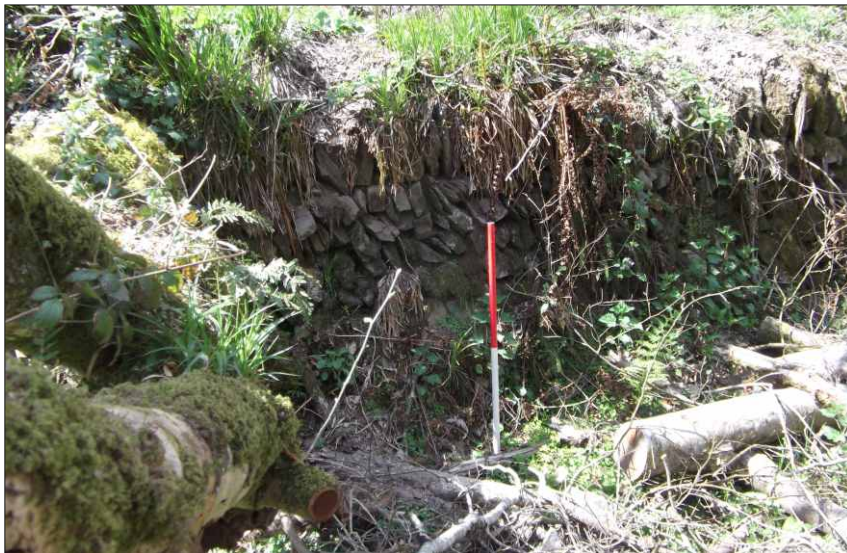
Plate 5: Remains of embanked approach to Old Bridge, looking northwest (1m scale)
