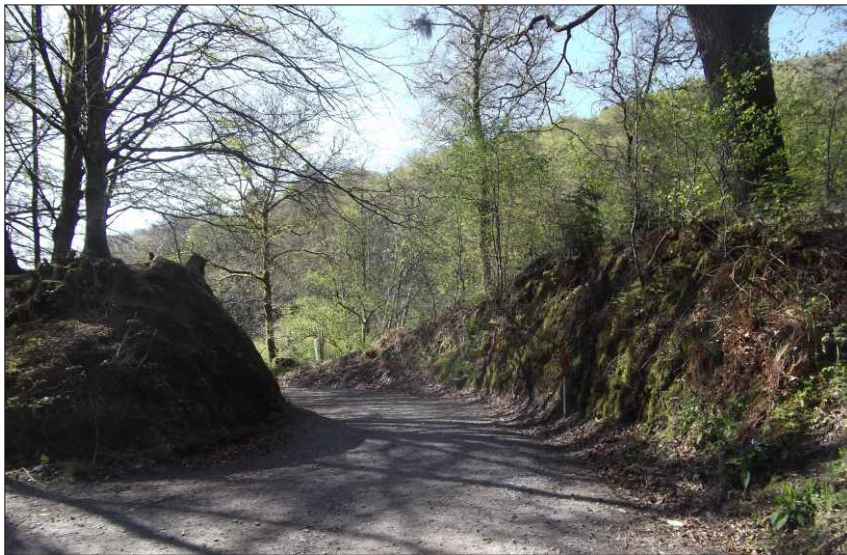
Plate 2: Lower carriageway to dam showing cutting close to Smallacombe Drive junction, looking southwest (1m scale)
