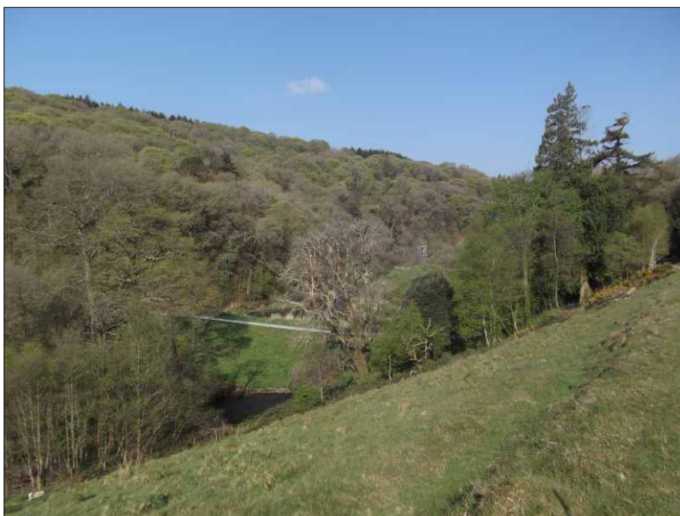
Plate 9: Views towards dam from Smallacombe Drive, looking northwest
