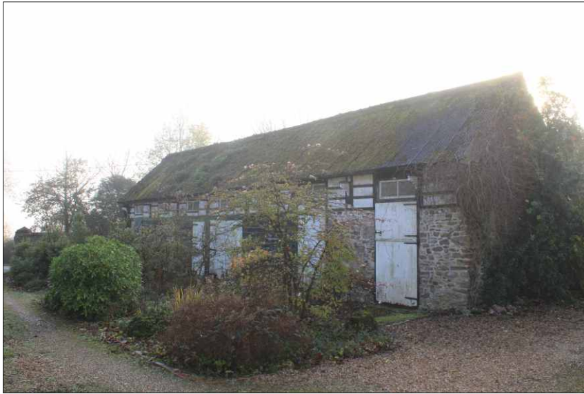
Plate 1: General view of the outbuilding, looking southeast
