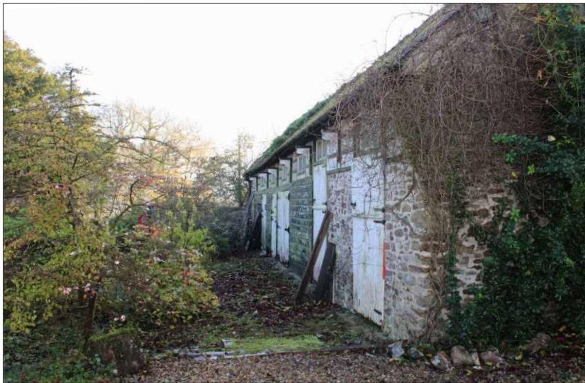
Plate 2: North elevation, looking east (1m scale)
