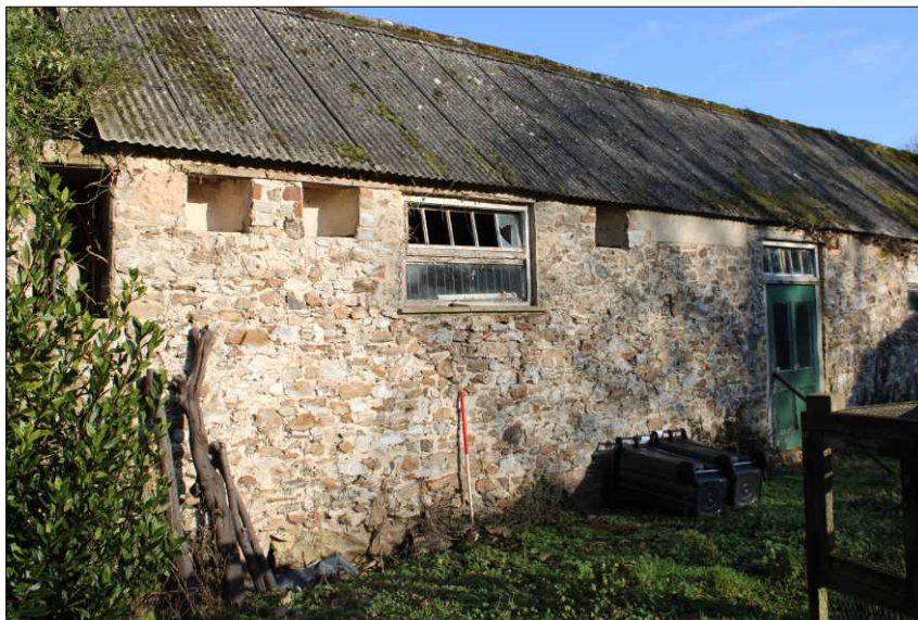
Plate 6: South elevation, looking northeast (1m scale)
