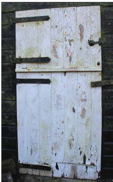
Plate 3: View of one of the stable doors showing the decorative fittings, looking south
