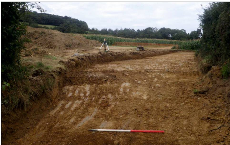
Plate 1: General view of monitored drive, looking northwest (scale 1m)
