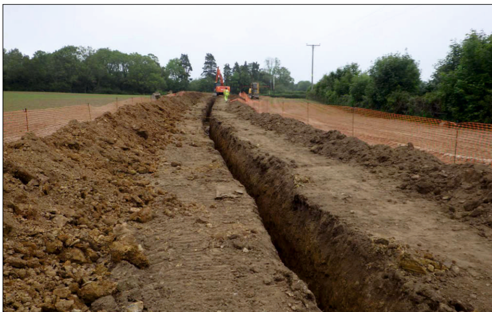
Plate 2: General view of cable trench, looking east
