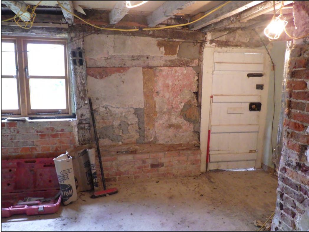
Plate 3: Primary framing in SE elevation (scale 1m)
