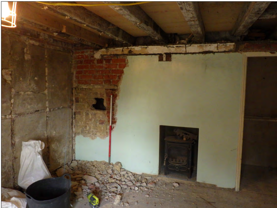
Plate 4: Period III inserted stack, latterly reduced in size with blocked alcove to left (scale 1m)
