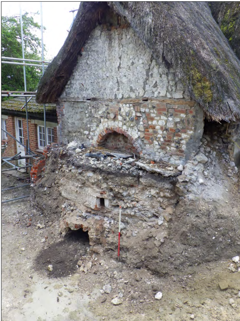
Plate 2: NW facing elevation of Oven 214 below Period III gable (scale 1m)
