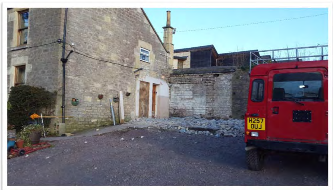
Plate 1: Area of the works prior to construction. View from the S
