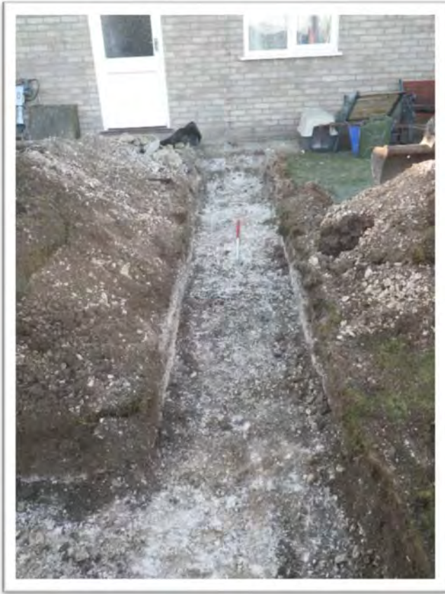
Plate 1: Footings trench from the northeast. 1m scale
