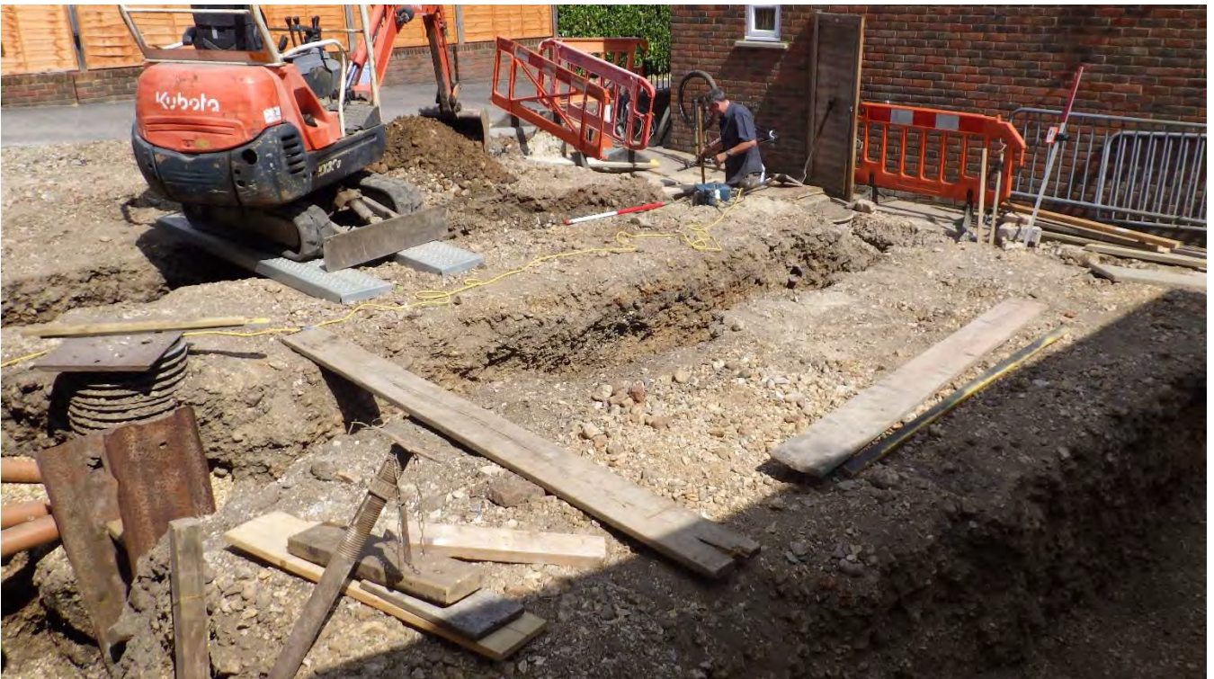
Plate 2: General view of building footings. View from the northwest. Scale 1m
